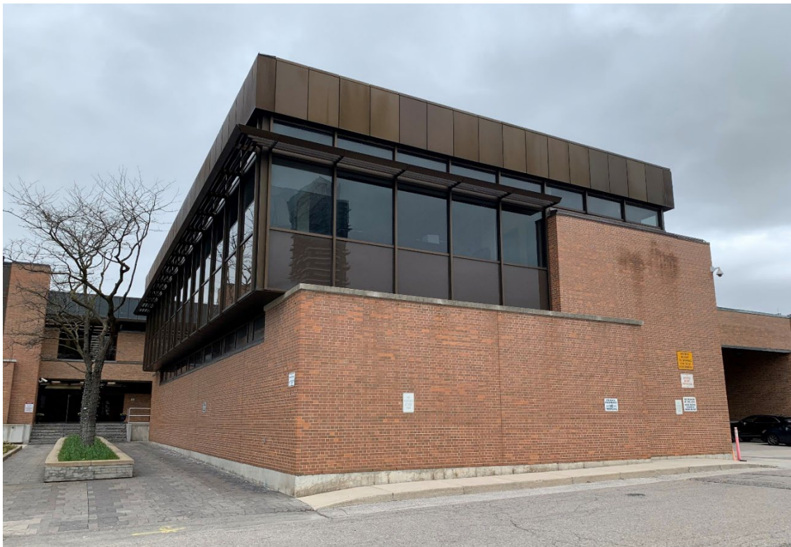
Figure 37. View of the south and west elevations of the southwest office addition, built in 2003-2004, looking north (Heritage Planning, 2023)
