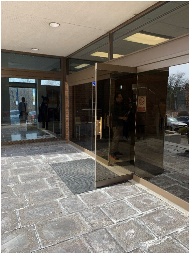
Figure 28. View of the primary entrance of the original 1962 office building showing the bronze doors, looking northwest (Heritage Planning, 2023)
