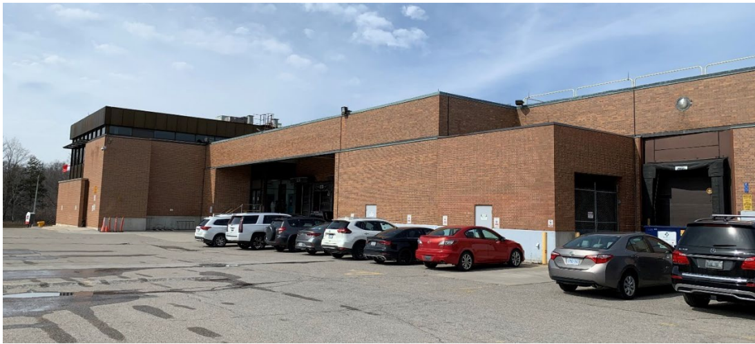
Figure 38. View of the south and east elevations of the southwest office addition (left) and the south elevation of the plant (right), looking northwest (Heritage Planning, 2023)
