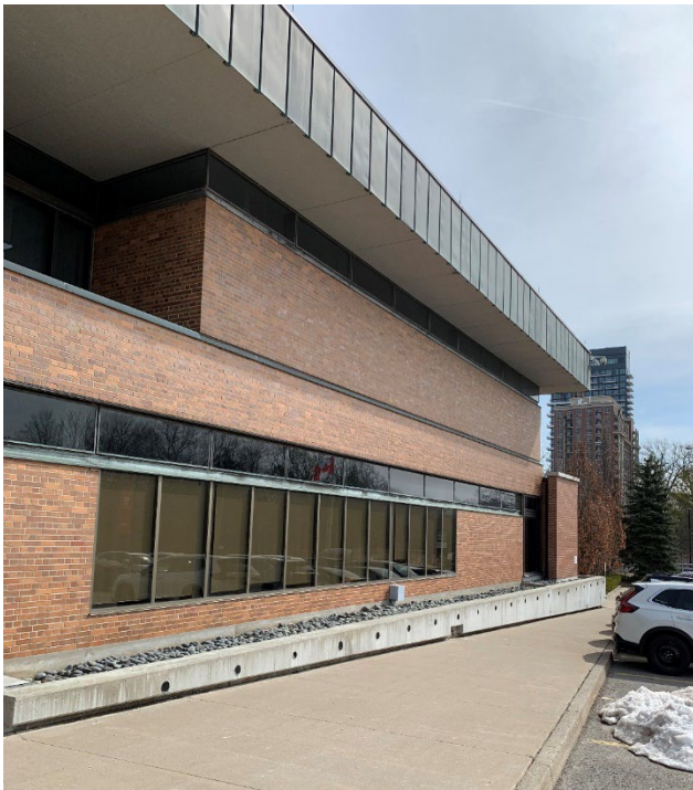
Figure 32. View of the west elevation of the original 1962 office building showing the new window openings added to the building as part of the 2003-2004 renovation and extension, looking south (Heritage Planning, 2023)
