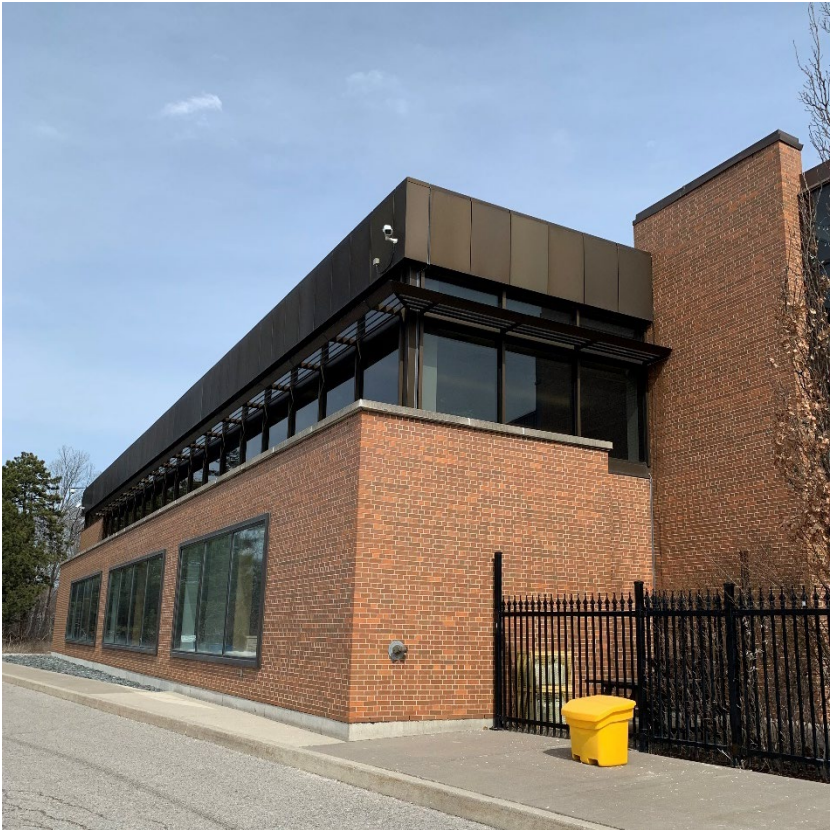
Figure 33. View of the south and west elevations of the northwest office addition, built in 2003-2004, looking northeast (Heritage Planning, 2023)
