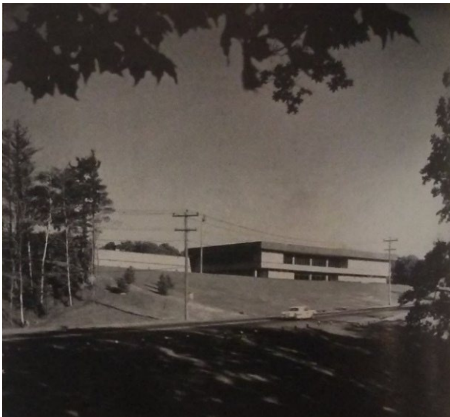
Figure 15. View of the north and west elevations from the west side of Leslie Street showing the original office building on the right and the plant on the left, looking southeast (RAIC Journal, Vol. 40, No. 7, July 1963)
