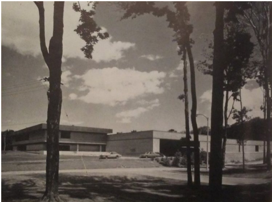
Figure 14. View of the south and west elevations from the neighbouring property showing the original office portion on the left and the plant on the right, looking northeast (RAIC Journal, Vol. 40, No. 7, July 1963)
