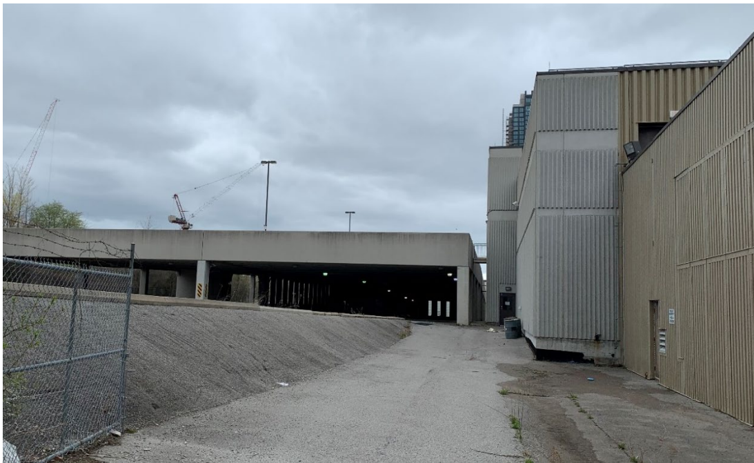
Figure 42. View of the two-storey parking garage (left) and the rear additions to the plant (right), looking south (Heritage Planning, 2023)
