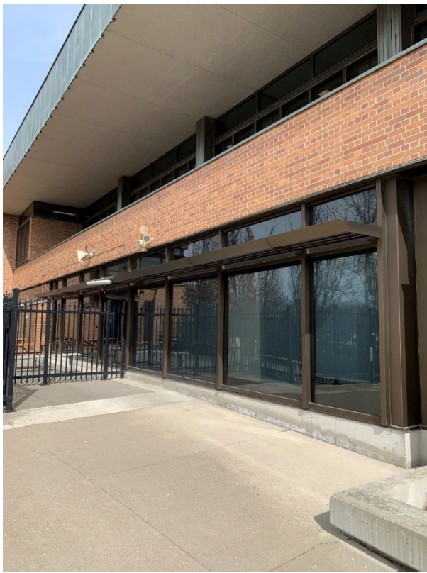
Figure 31. West elevation of the original 1962 office building showing the new windows on the first floor (as part of the 2003-2004 extension/renovation) and the original recessed area on the second floor, looking north (Heritage Planning, 2023)
