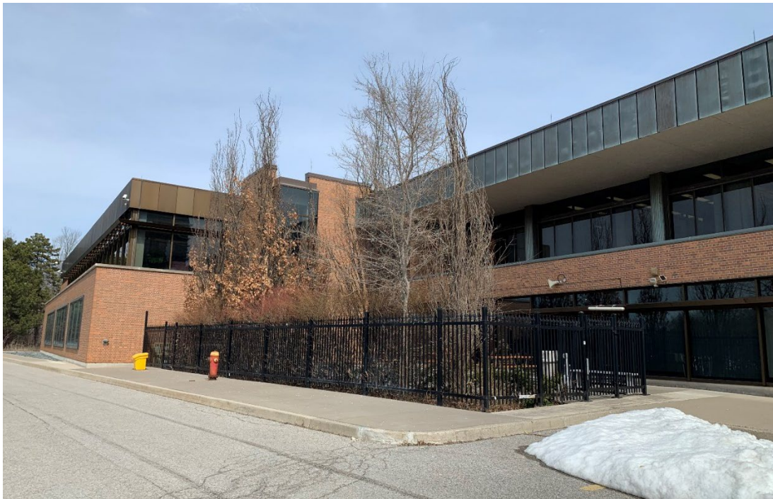
Figure 34. View of the west elevation of the original 1962 office building (right) and the south and west elevations of the northwest office addition, constructed in 2003-2004 (left) showing the enclosed courtyard located between the surface parking and the office buildings, looking northeast (Heritage Planning, 2023)
