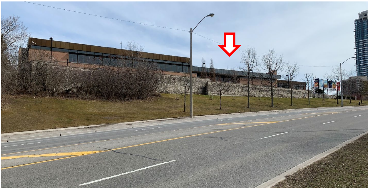
Figure 23. 1123 Leslie Street: west elevation of the former William Wrigley Jr. Company complex showing the raised landscape setting and the stone retaining wall, looking southeast; the red arrow indicates the location of the original 1962 office building (Heritage Planning, 2023)
