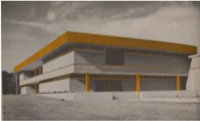
Figure 9. Photograph of the west and south elevations of the original office building; the photo highlights where the bronze metal cladding is located on the building, as part of an Anaconda metals advertisement (RAIC Journal, Vol. 40, No.7, July 1963)
