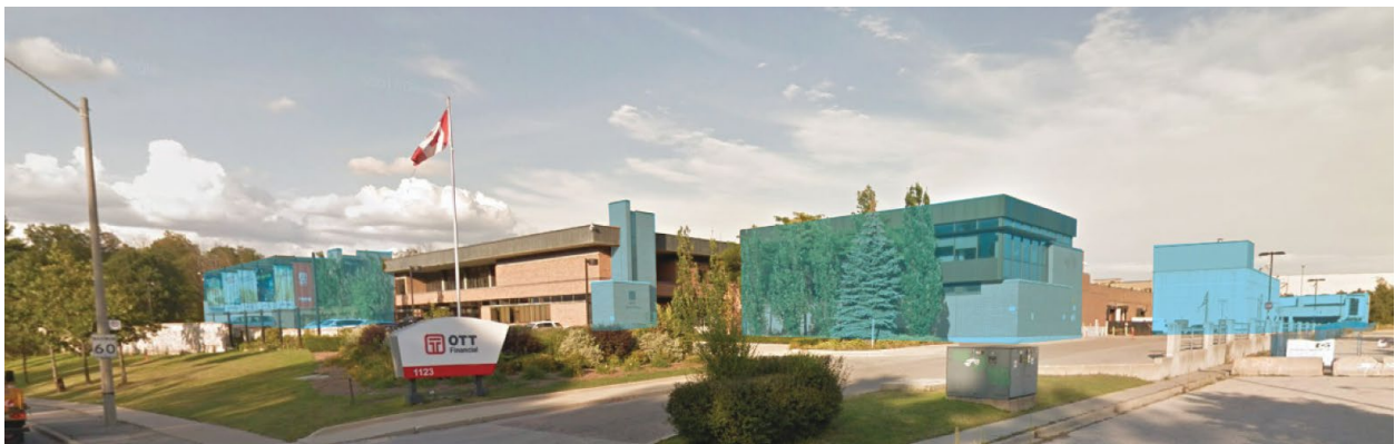
Figure 8. Photograph of the subject property at 1123 Leslie Street indicating in blue the parts of the complex added between 2002-2007 (ASI, p. A-5)
