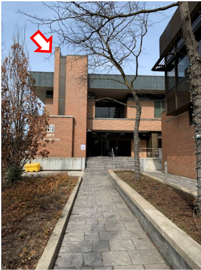
Figure 24. South elevation of the original 1962 office building showing the elevator shaft added to the original office building (marked by the red arrow) and the landscape features including the planter and trees on the south side of the primary entrance, looking north (Heritage Planning, 2023)
