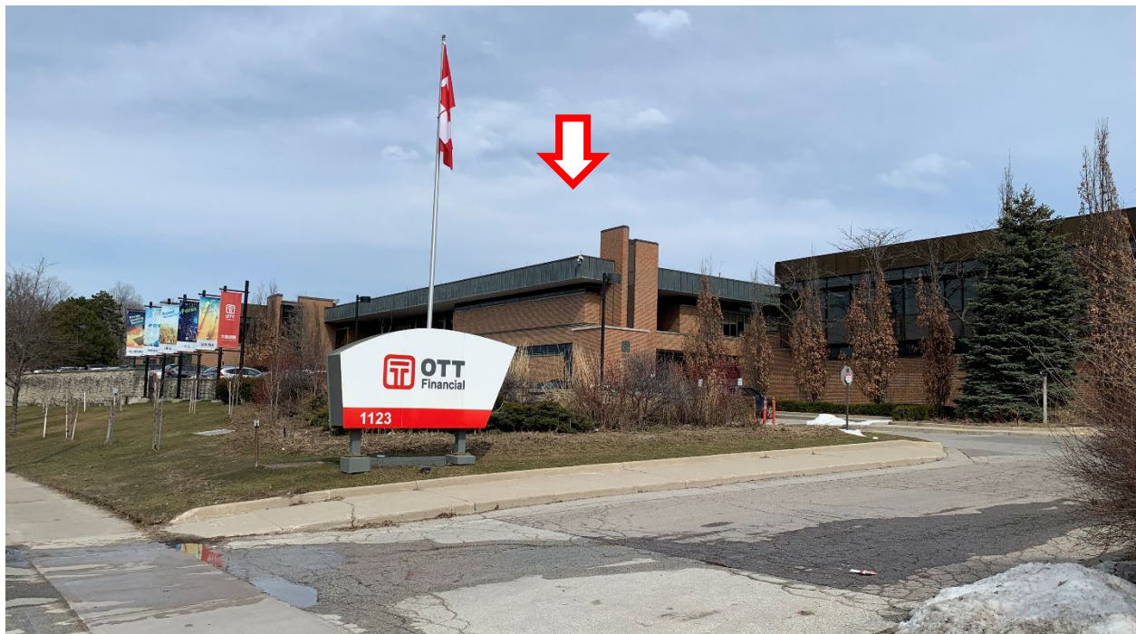
Figure 21. View of the office portion of the former William Wrigley Jr. Company complex showing the original office building constructed in 1962, marked by the red arrow, looking northeast (Heritage Planning, 2023)
