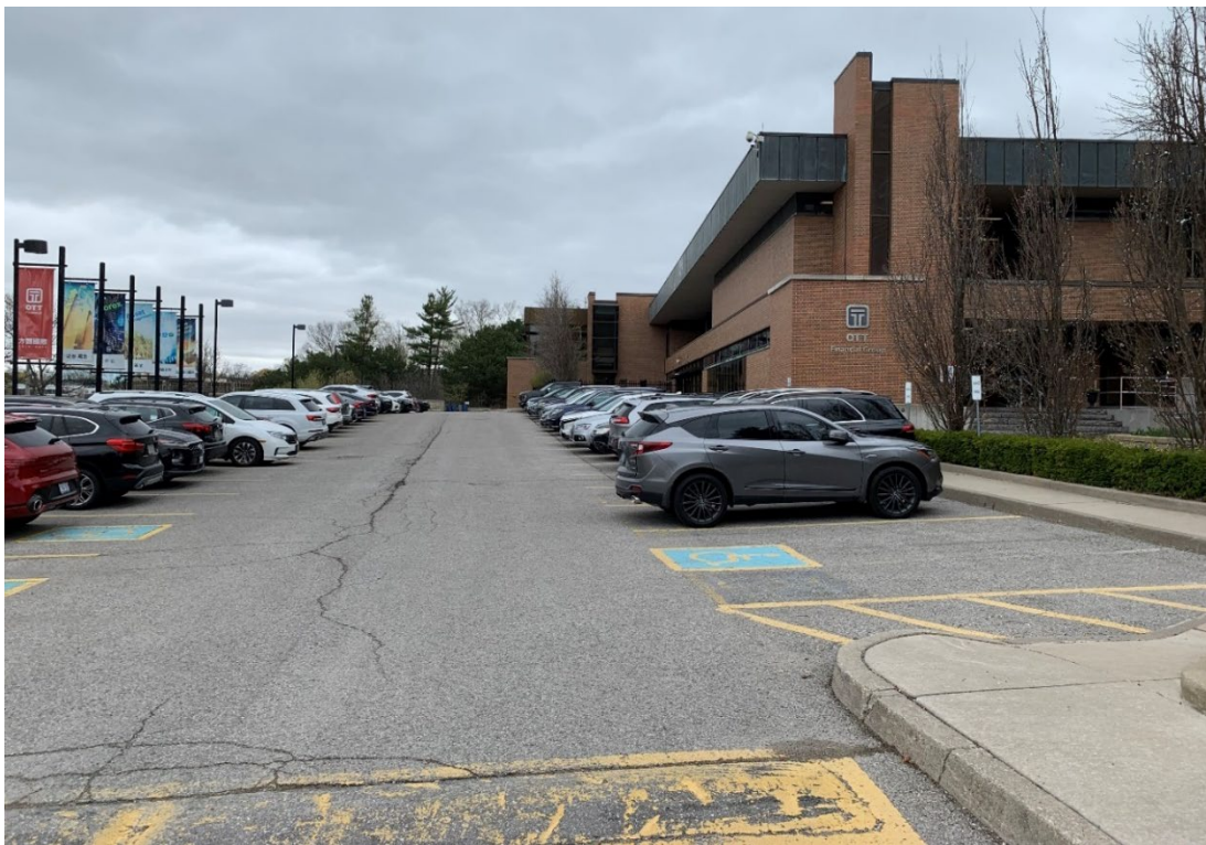
Figure 35. View of the south and west elevations of the original 1962 office building, south elevation of the northwest office addition, and the surface parking facing Leslie Street, looking north (Heritage Planning, 2023)
