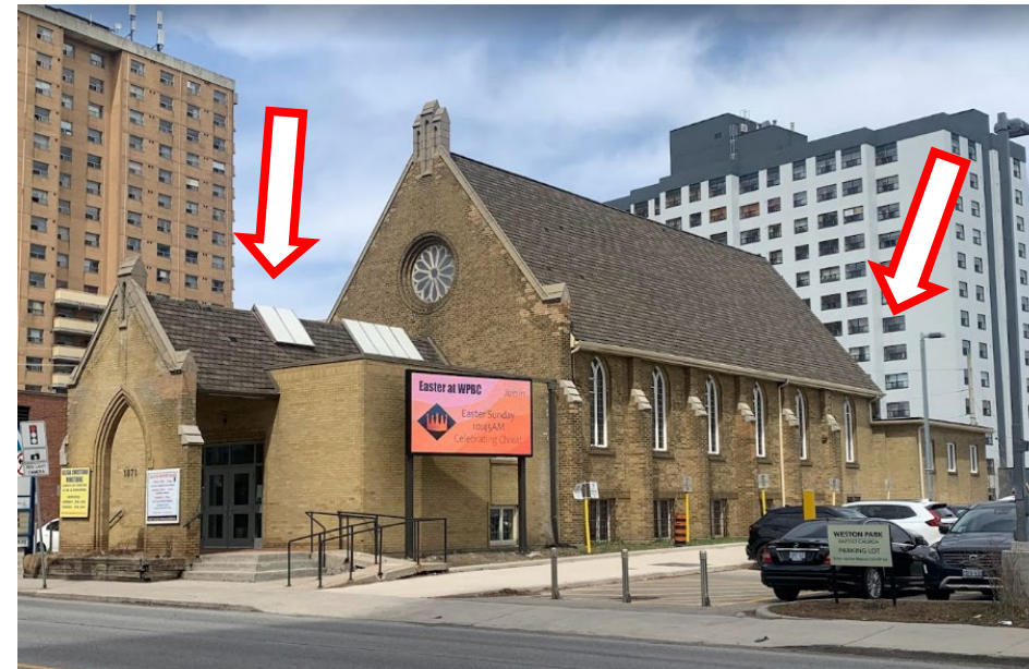
Current photo showing the west and rear (east) alterations
