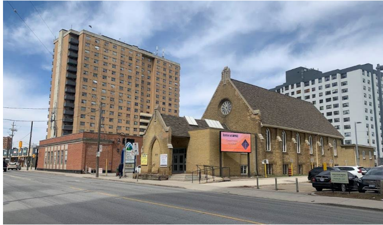
Looking northeast at the site
