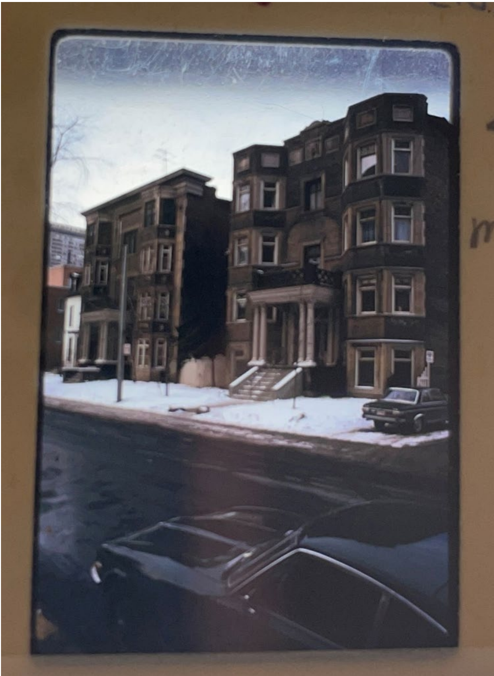
Figure 4: The Maitlands, 1974 (Heritage Impact Assessment, LHC Planning and Architecture, December 22, 2022 from original at City of Toronto Archives, 42 Maitland Street, Fonds 2043, series 2523, File 848)
