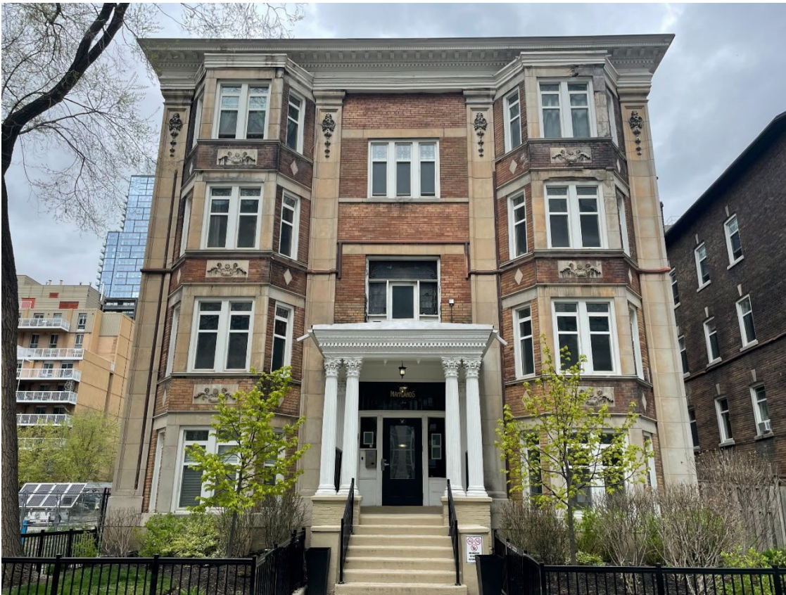
Figure 5: South (main) façade of 36 Maitland Street, 2023 (Heritage Planning)
