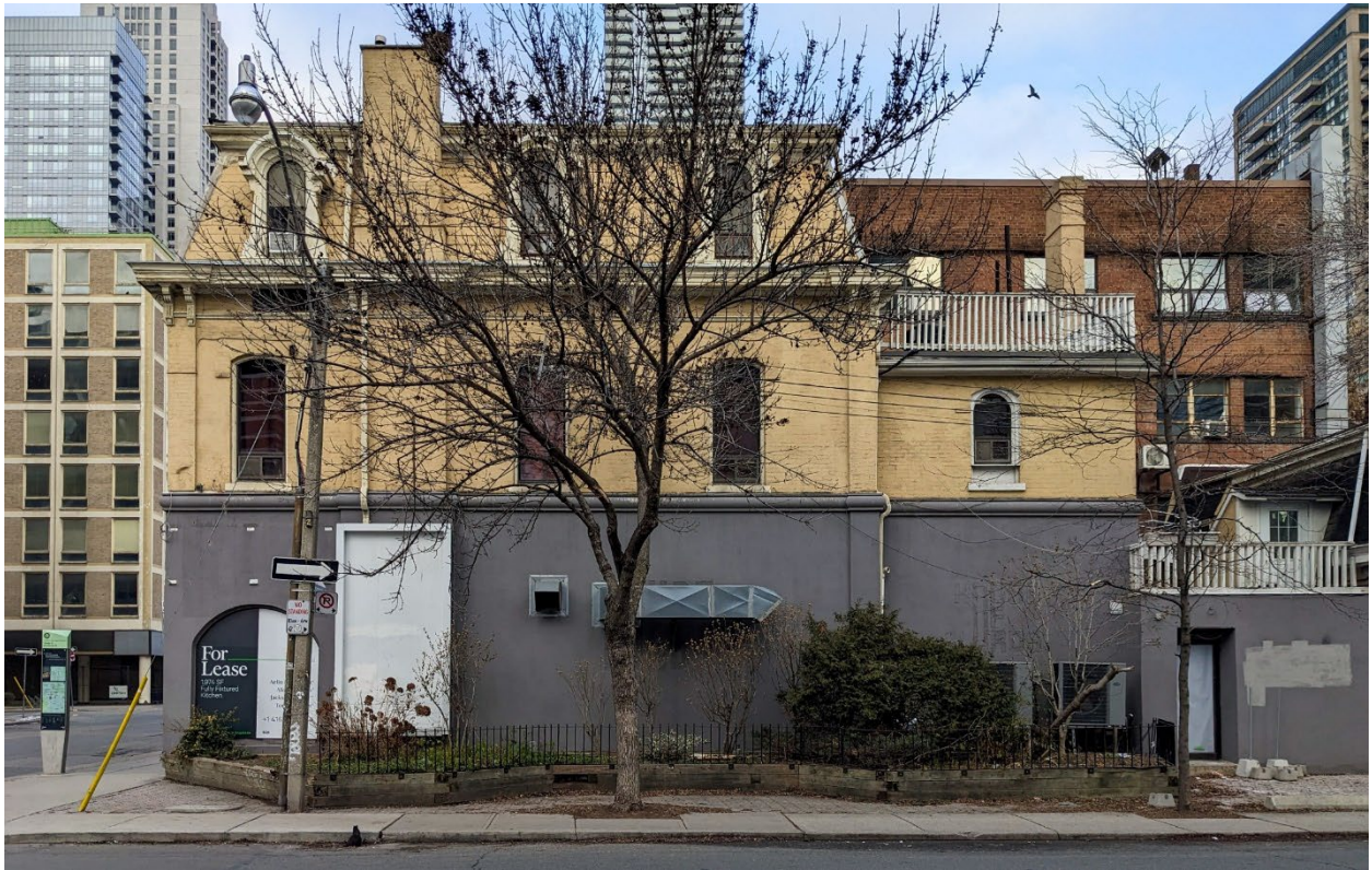
Figure 15. Partial south elevation of 639 Yonge Street, showing the primary structure and middle volume. A partial south elevation of 641 Yonge Street is visible beyond (Heritage Planning, 2022).
