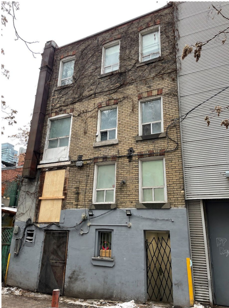
Figure 22. East elevation of the rear warehouse building on 649 Yonge Street (Heritage Planning, 2022).
