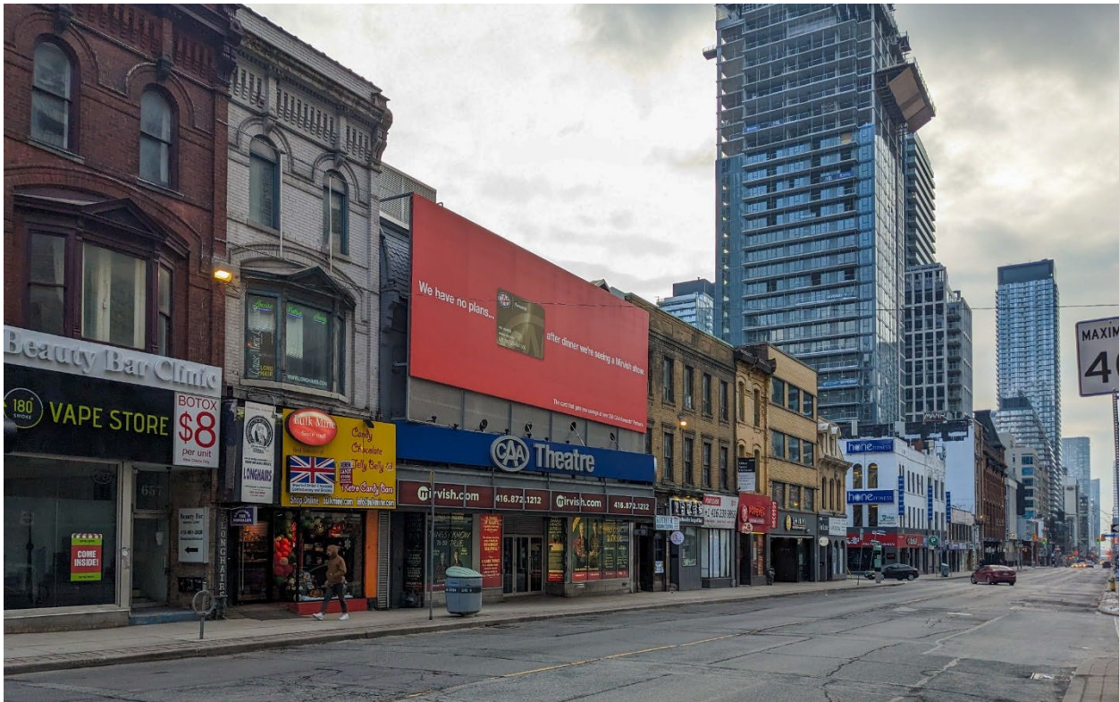
Figure 26. View of 639-651 Yonge Street looking southeast along Yonge Street (Heritage Planning, 2022).
