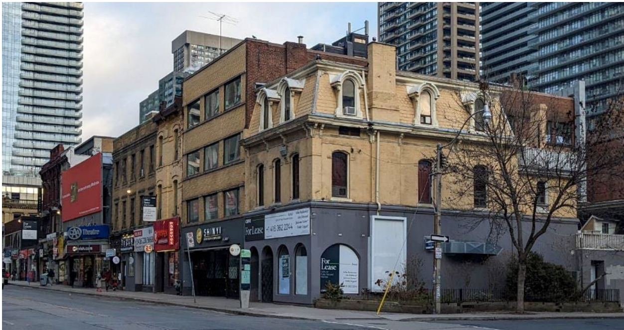
View of the subject properties from the southwest, with 639 Yonge Street in the foreground (Heritage Planning, 2022)
