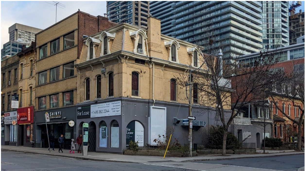
Figure 13. West and south elevations of 639 Yonge Street (Heritage Planning, 2022).
