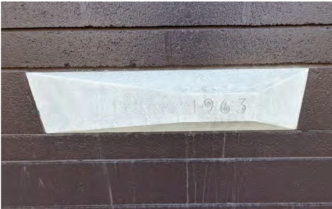
37. Current photo showing the date stone with "1963" located next to the main entrance on the north elevation, 2023 (Heritage Planning)
