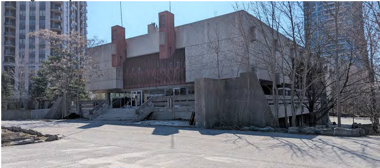
View of the subject property at 123 Wynford Drive, showing the west (principal) and south elevations of the former Japanese Canadian Cultural Centre (Heritage Planning, 2023).
