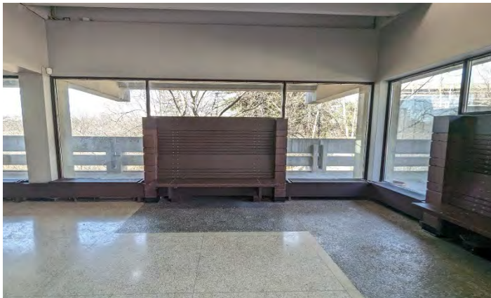
59. Current photo showing the bench seating in the lobby and polished terrazzo flooring with exposed pea gravel finish detailing, 2023 (Heritage Planning)
