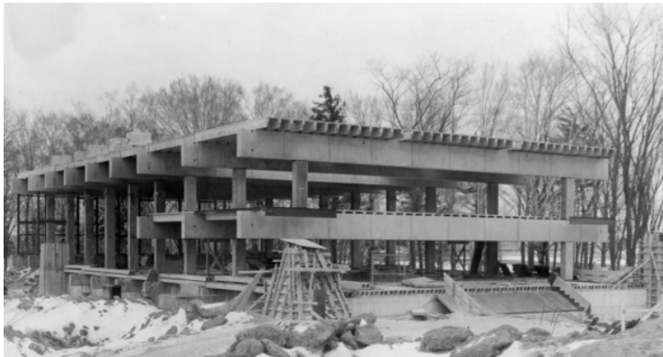
26. JCCC building under construction, structural elements, 1963 (JCCC Archives)
