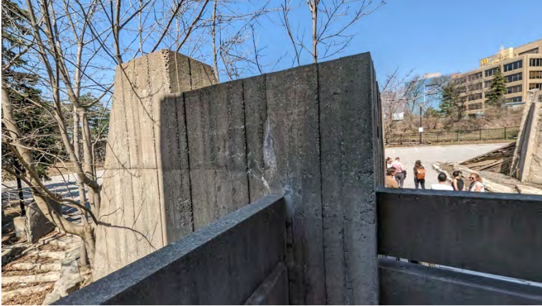
29. Concrete pylon at the northwest corner of the building, 2023 (Heritage Planning)
