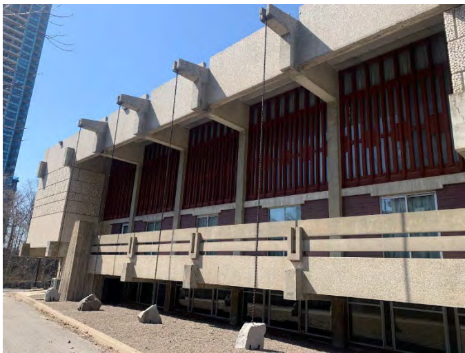
39. Current photo showing the east elevation, 2023 (Heritage Planning)
