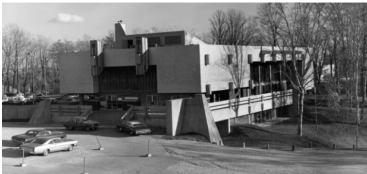
27. Completed JCCC building but prior to commencing landscaping, 1964-1975 (JCCC Archives)
