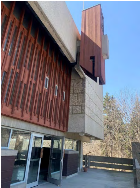
34. Current photo showing a detail of the wooden screen and west lantern on the north elevation, 2023 (Heritage Planning)
