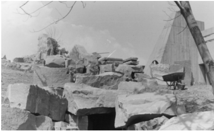
70. Archival photo of the landscaping under construction. Note the massive concrete pylon at right, 1964-1975 (JCCC Archives)
