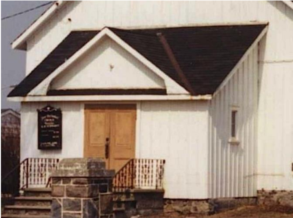
Replacement of front entrance door
