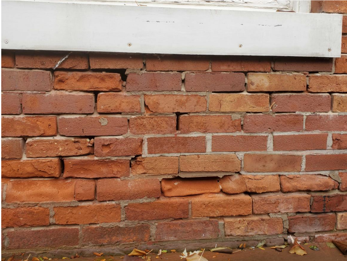
Small scale masonry repair and restoration – 134 First Avenue (Riverdale HCD)
