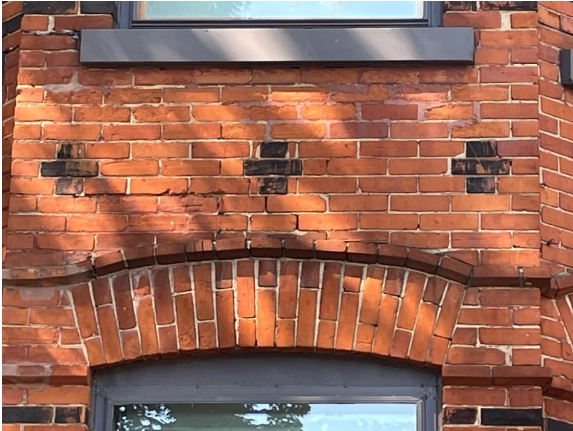
Small scale masonry repair and restoration – 46 Rose Avenue (Cabbagetown Northwest HCD)
