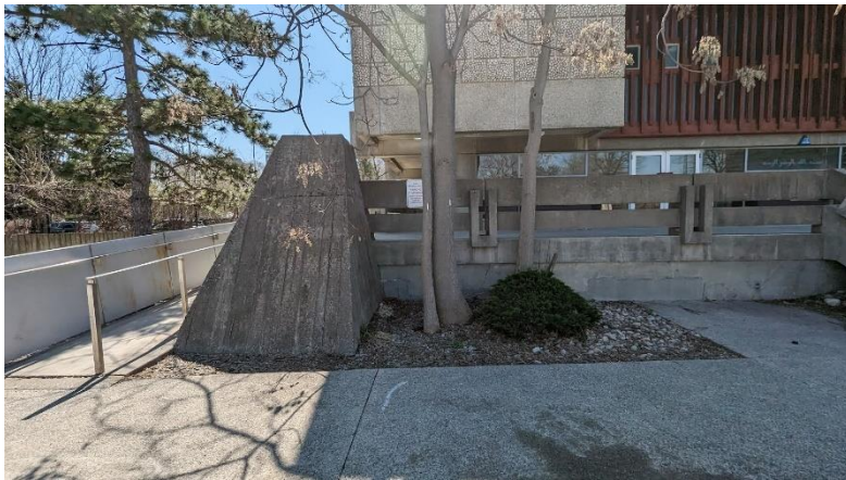
Northeast concrete pylon, 2023
