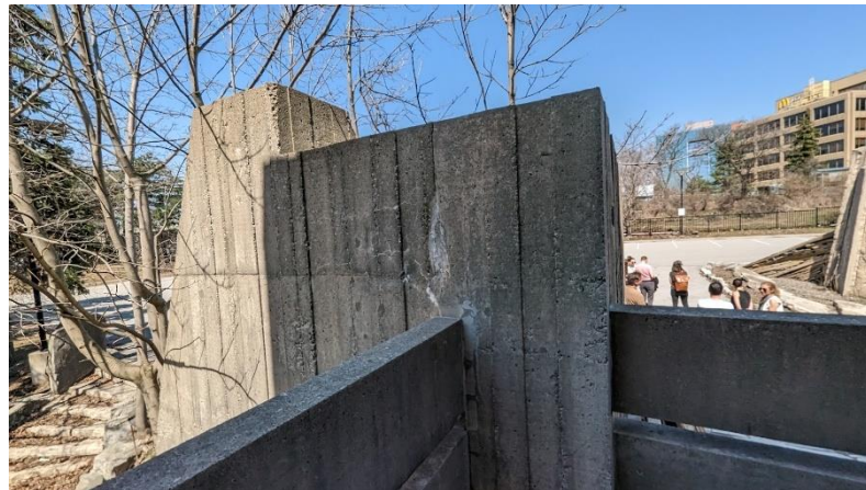
Northwest concrete pylon, 2023
