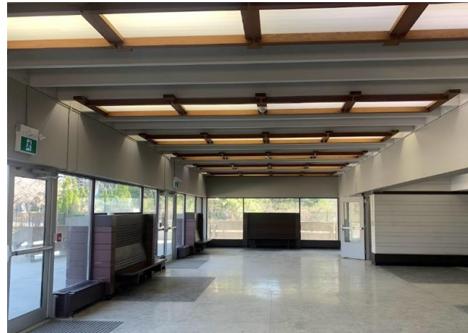
Main Floor (lobby)
