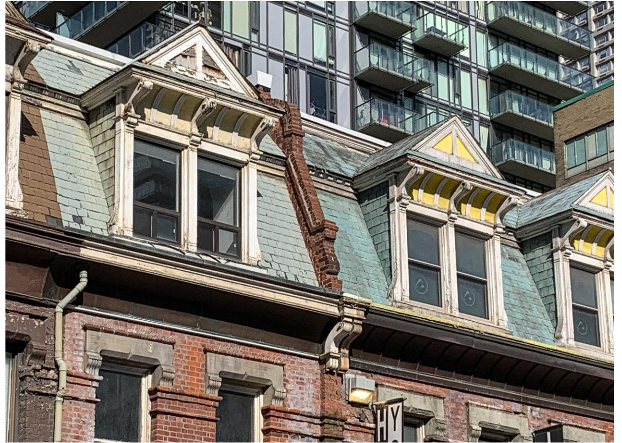
Detail of dormers, 678-680 Yonge Street (Heritage Planning 2023)
