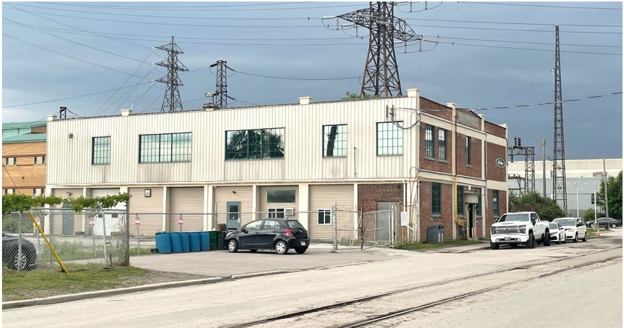
Figure 15. Context view looking west. Heritage Planning, 2023.
