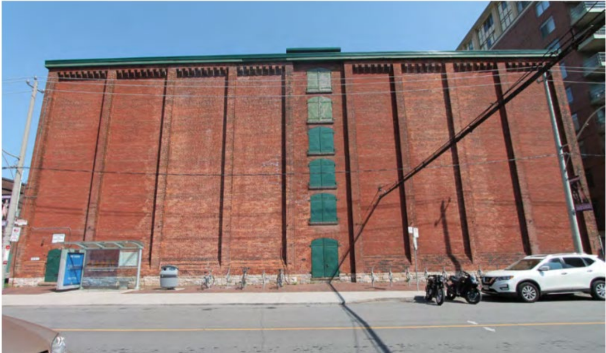
60 Mill Street, south elevation of Rack House D. (ERA Architects Inc.)
