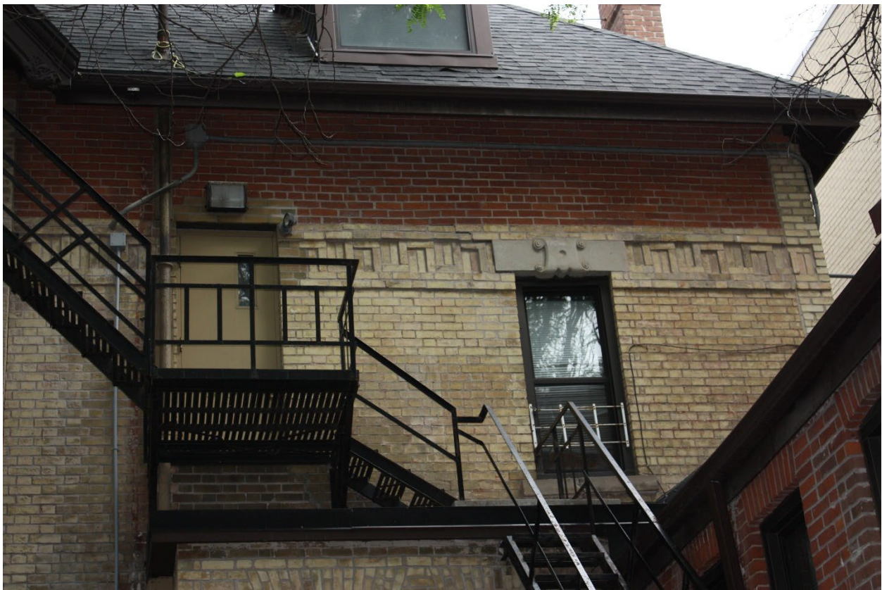
Figure 29. Detail of brick string course on south elevation of 137 Bond Street (Heritage Planning, 2023).
