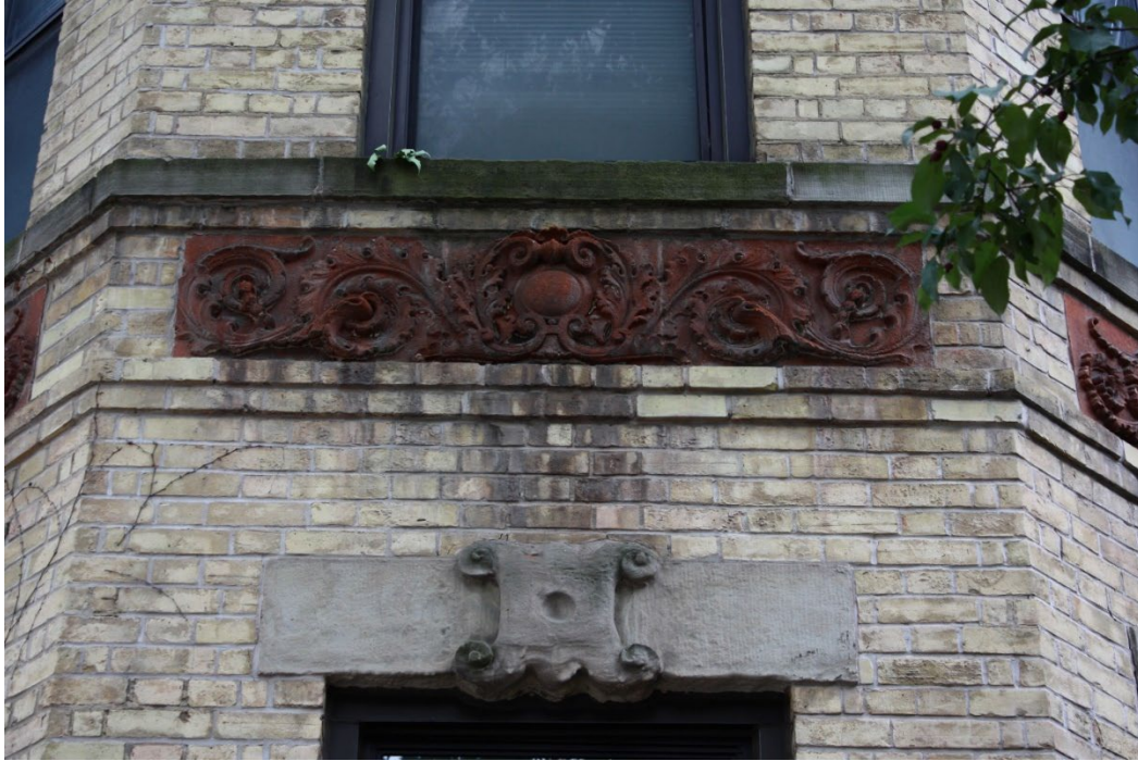
Figure 28. Detail of terracotta panel on turret of 137 Bond Street (Heritage Planning, 2023).
