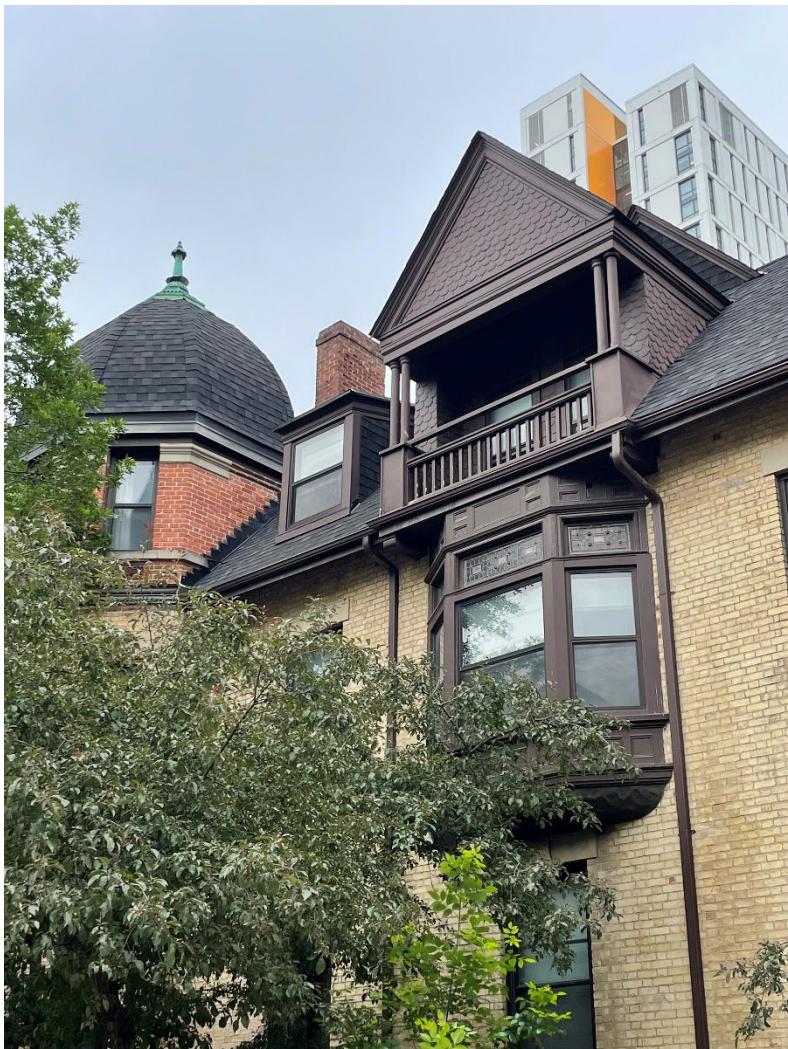
Figure 31. Detail of the north elevation oriel window, balcony, wall gable, and turret (Heritage Planning, 2023).
