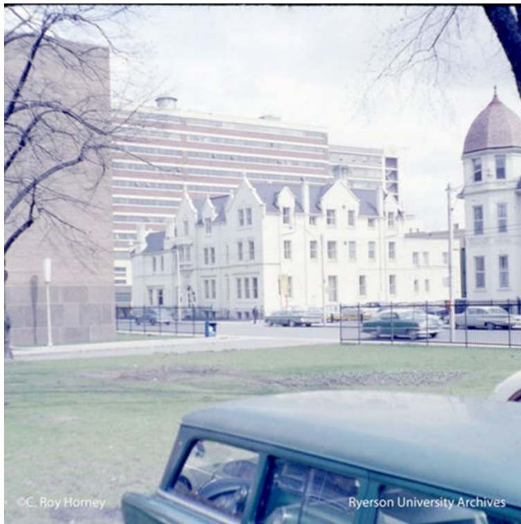
Figure 13. "Oakham House", 1961 Turret of 137 Bond Street shown with painted masonry (paint removed by 1976). photograph by Charles Roy Horney (TMU Archives, item F 536.16.05).
