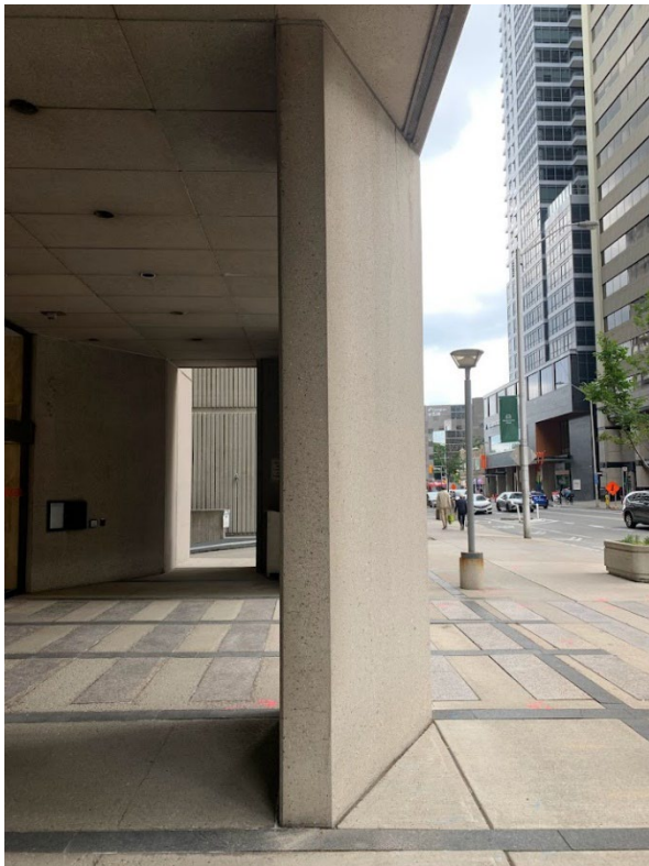
Image 37. Current photograph of a pre-cast concrete perimeter column on the east elevation (Heritage Planning, 2023)
