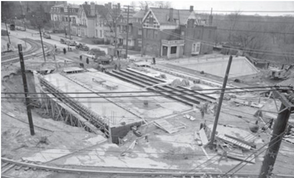
Image 10. 1946 aerial photograph looking northwest at construction of the Bloor Street underpass and Clifton Road Extension, later renamed Mount Pleasant Road, from south of Bloor Street East (Toronto Public Library).
