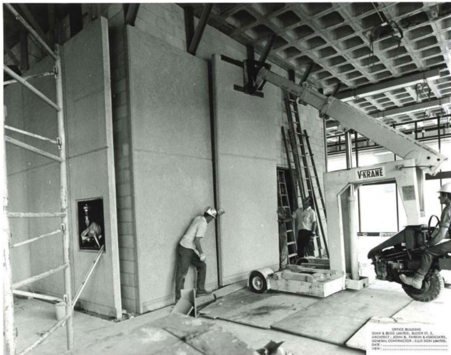
Image 28. 1969 photograph of the building interior during installation of concrete panels. Also visible is the waffle form of the second-storey concrete floor slab above (Panda Associates).
