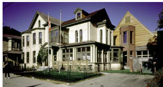
1990s photograph of 291-295 Sherbourne Street, showing original historic building fabric retained (left) and a portion of the infill volume (right) (Hariri Pontarini).
