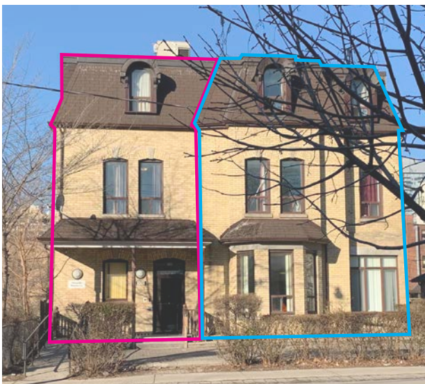
2023 east elevation of 300 Sherbourne Street (ERA, 2021).
