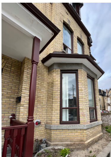
East elevation bay with stone lintels and sills original building (ERA, 2023).
