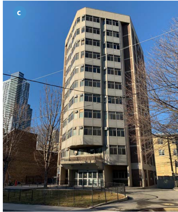
Existing 1970s 11-storey tower residences at 100 Pembroke Street, just west of the Site (constructed 1976, unknown architect.) (ERA, 2021).
