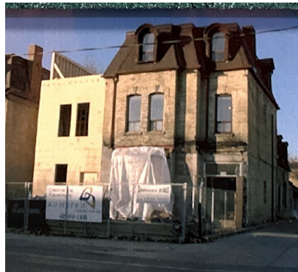
East elevation of 300 Sherbourne during the 2004 construction (Kennedy Residence).
