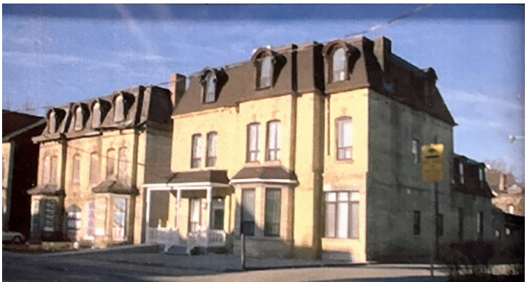
2004 post construction (Kennedy Residence).
