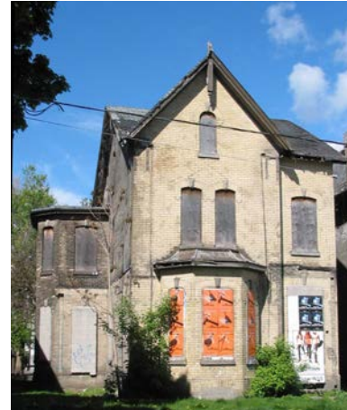
Former John H. Thom House at 294 Sherbourne Street (Bob Krawczyk, Architectural Conservancy of Ontario).
