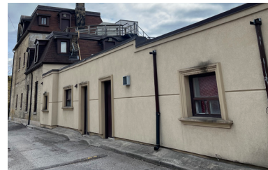
North elevation of the non-original stucco wing (ERA, 2023).
