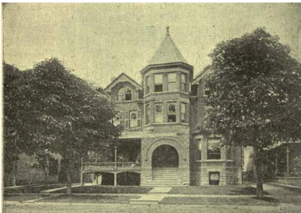
1894 photograph of the former Toronto College of Music at 12-14 Pembroke, demonstrating the prominent architecture and lush landscape of this Street (Toronto Public Library).
