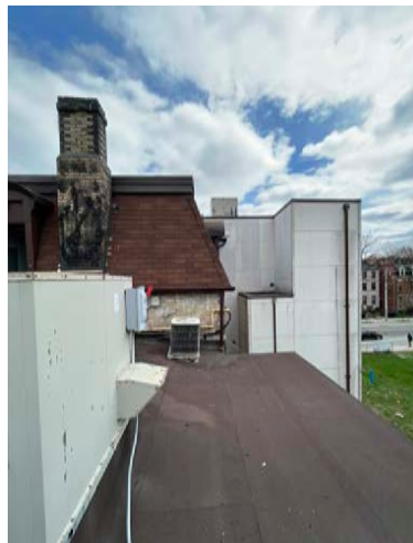
View east from one-storey stucco wing towards the west (rear) elevation of the original building (left) and addition (right) (ERA, 2023).
