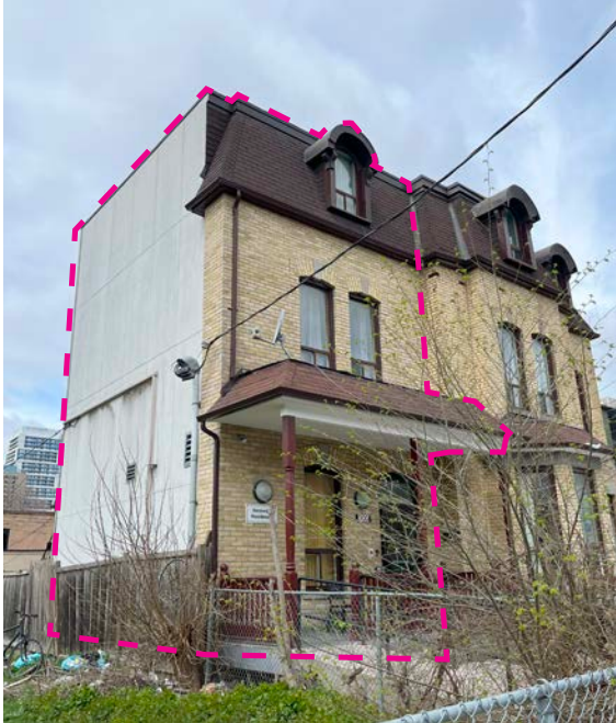
South and east elevation (ERA, 2023).
