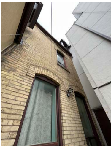
View of south and east elevation interface between original building (left) and addition (right) (ERA, 2023).
