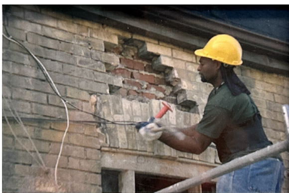
2004 construction at 300 Sherbourne Street (Kennedy Residence).
