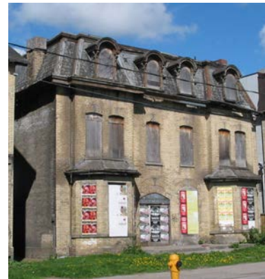
Former semi-detached house at 296-298 Sherbourne Street (Bob Krawczyk, Architectural Conservancy of Ontario).
