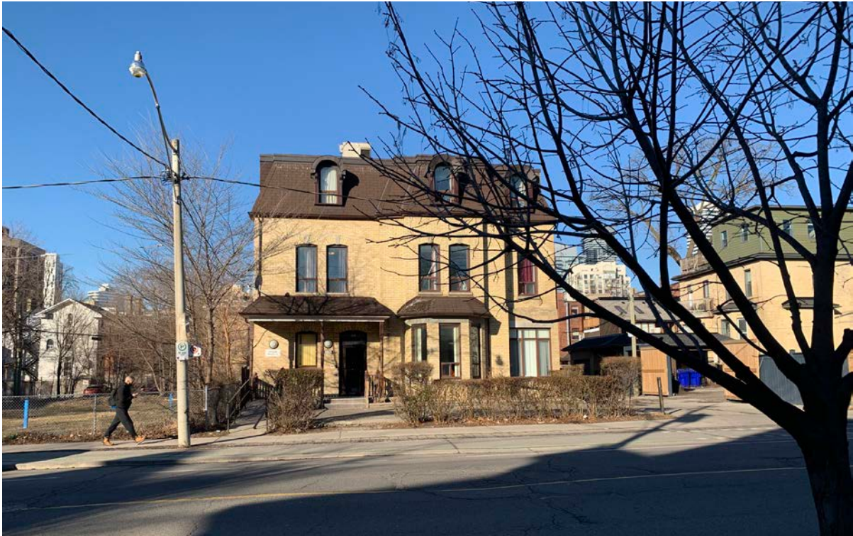
View of the east elevation of 300 Sherbourne Street on the Site (ERA, 2021).
