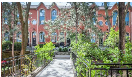
280 Sherbourne Street, units 1-4. This 1979 infill project was designed by Ferdinand A. Wagner in a late modernist style. It is flanked by two 19th century houses to the north and south. (Top: ACO, Bob Krawczyk, Bottom: Zolo).
