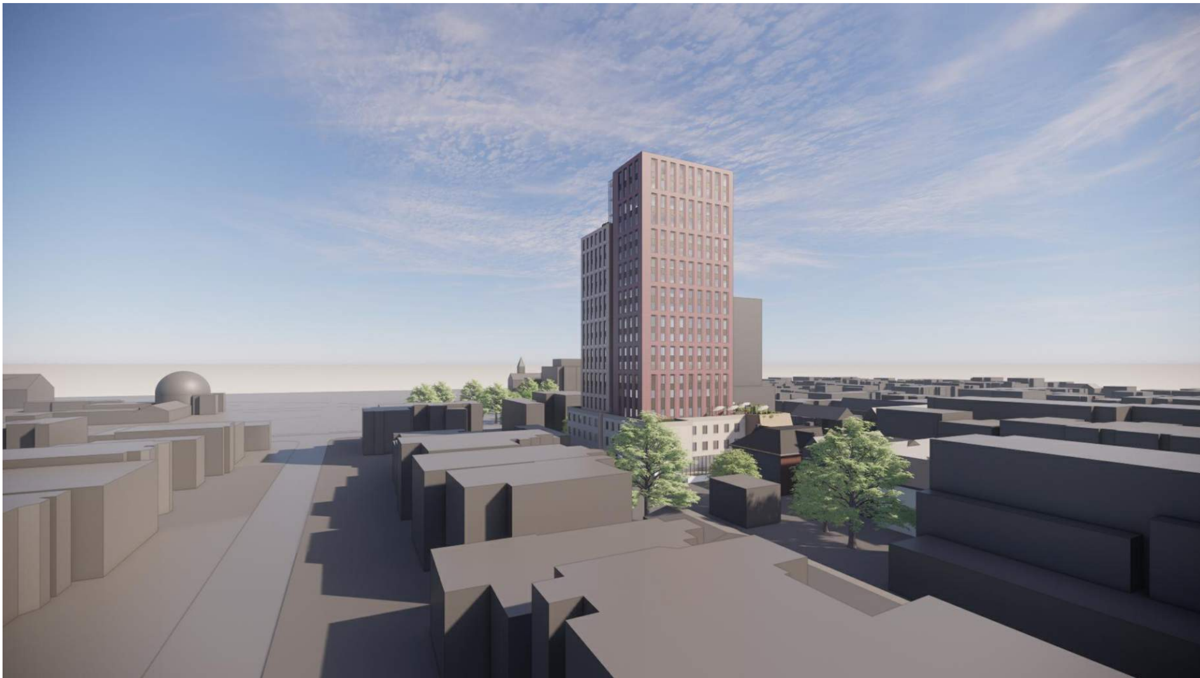
SOUTH WEST AERIAL VIEW FROM PEMBROKE ST.
