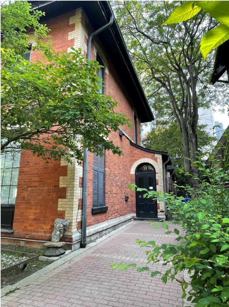
Above: 37 Maitland St., West façade showing main entrance, 2023 (Heritage Planning)
