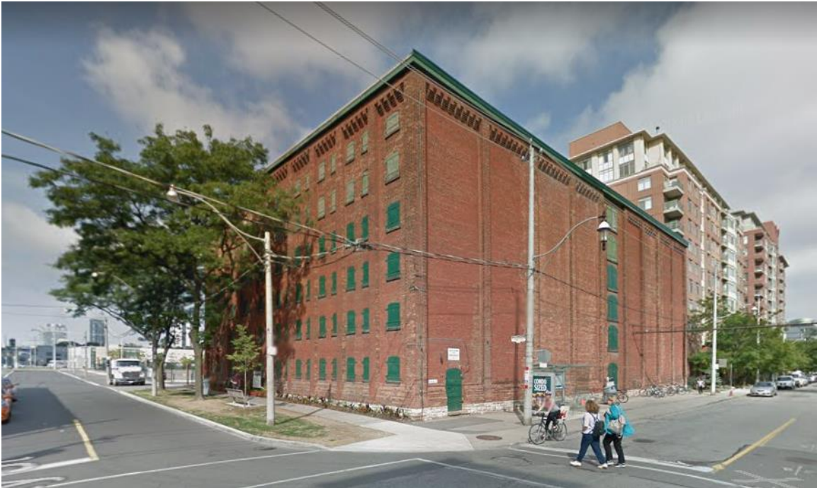
60 Mill Street South and West Elevations
