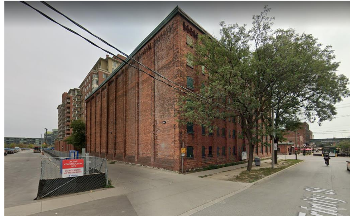
60 Mill Street North and West Elevations
