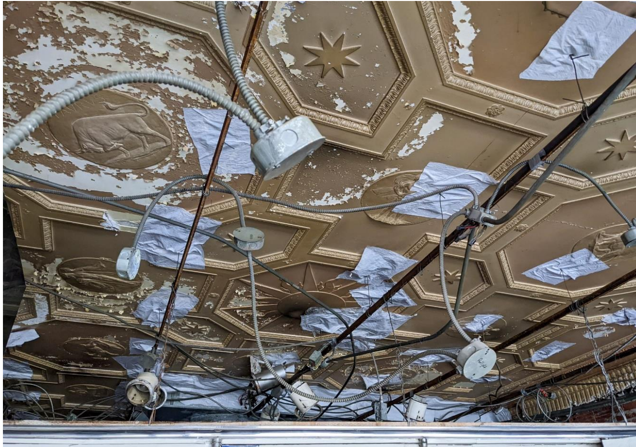
Partial lobby ceiling previously concealed (Heritage Planning, 2022)
