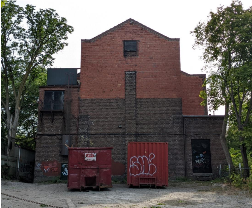
Rear (east) elevation (Heritage Planning, 2022)
