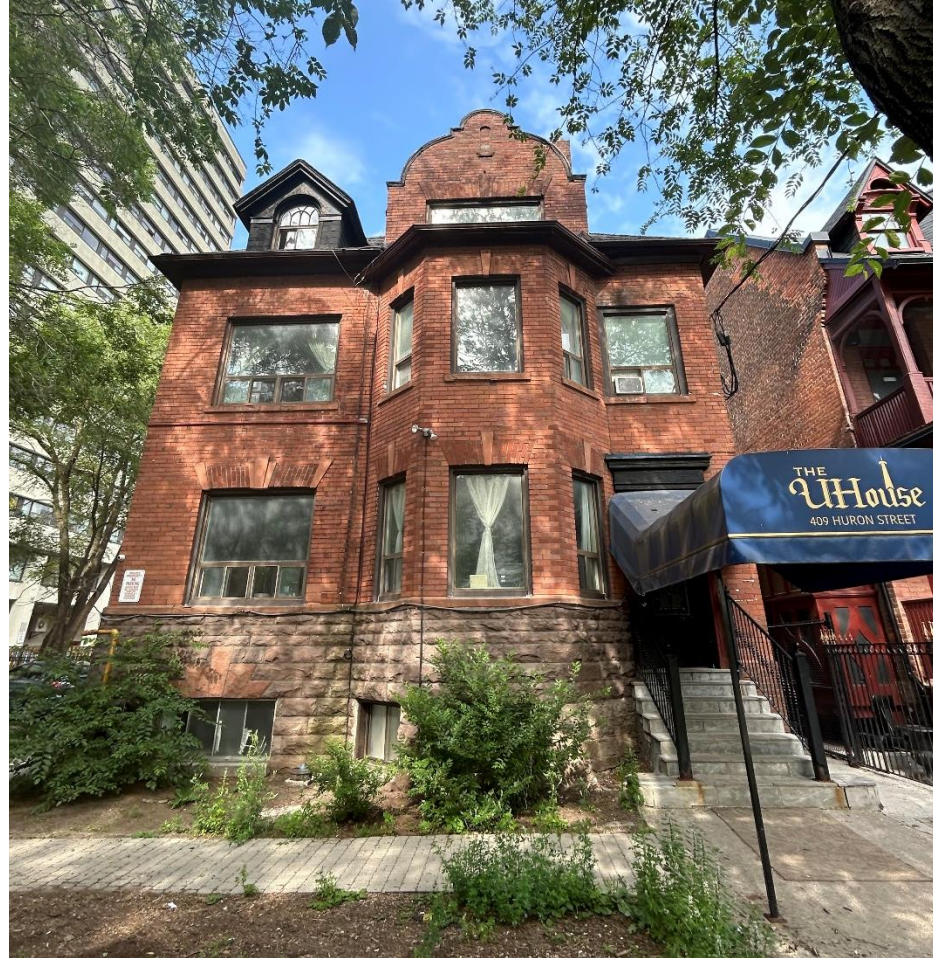
West elevation, 2023 (Heritage Planning).
