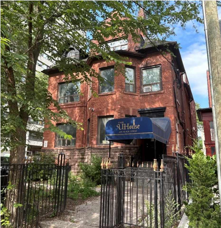
West elevation, 2023 (Heritage Planning).
