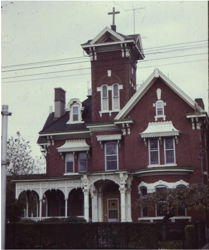
25 Augusta Avenue in 1970 (Toronto Historical Board slides).
