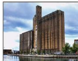
Canada Malting Silos
