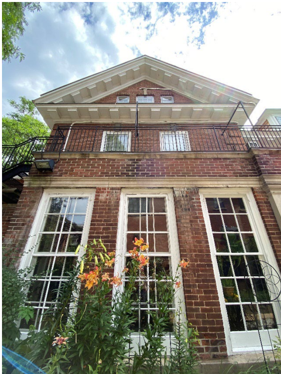
Figure 14. West elevation showing elongated window bays, dentils on gable end, and symmetry (Heritage Planning, 2023)
