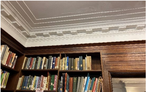
Figure 19. Dentils on covered ceiling. (Heritage Planning, 2023)
