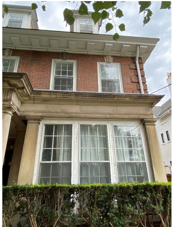
Figure 11. Triple window bay with Tuscan Doric pilasters to the right of the columned main entrance portico. (Heritage Planning, 2023)
