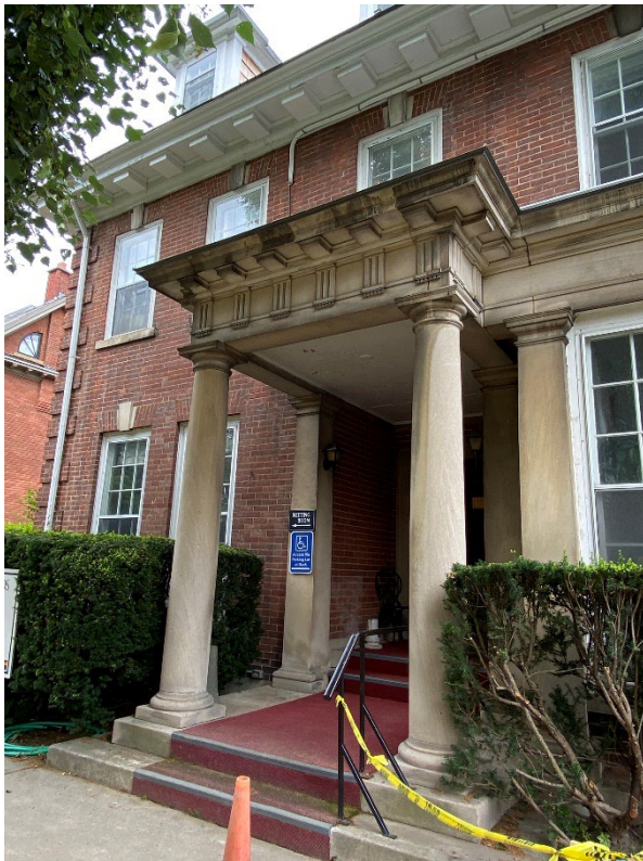
Figure 10. Main entrance portico on the south elevation with Tuscan Doric columns and entablature. (Heritage Planning, 2023)
