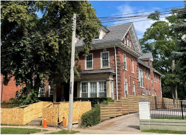
Figure 16. South and east elevations. (Heritage Planning, 2023)
