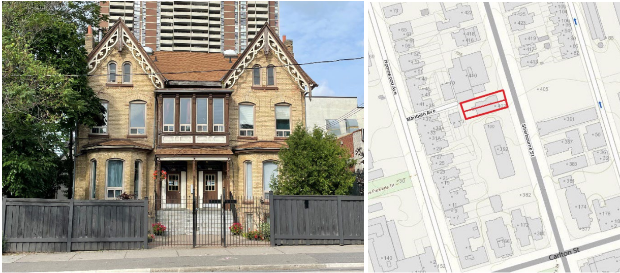
(Left) Front façade of 402 (left) and 404 (right) Sherbourne Street, Heritage Planning, 2023. (Right) Map of the area and 402 and 404 Sherbourne Street (indicated in red). Note: This location map is for information purposes only; the exact boundaries of the property are not shown. City of Toronto Mapping.
