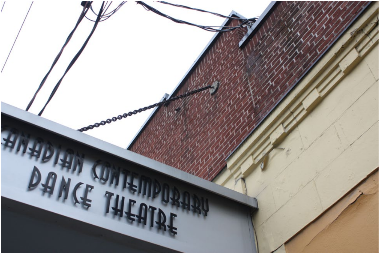
Figure 6. Detail of dentils, marquee, and marquee anchor on 509 Parliament Street, 2023 (Heritage Planning).
