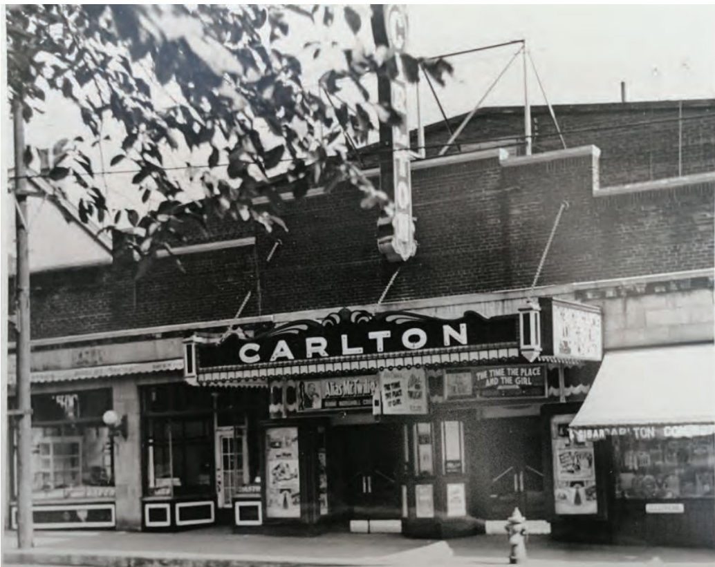
Figure 6. Historic image of the main façade (west) of 509 Parliament Street with its marquee and storefronts (since infilled), c.1937 (City of Toronto Archives).
