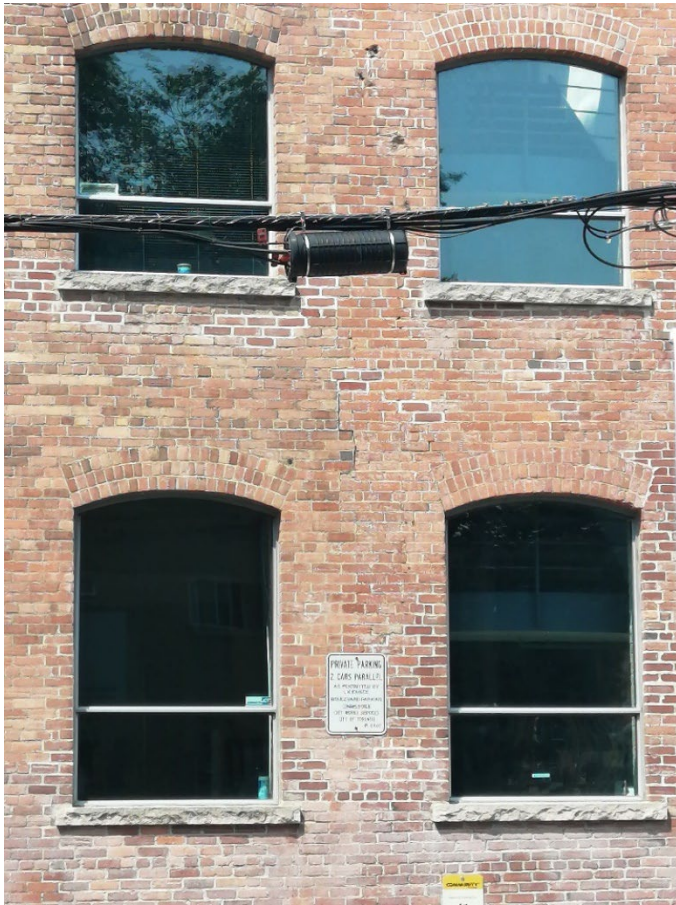
Figure 17: Close up of primary elevation with running masonry joints (Heritage Planning, 2023).
