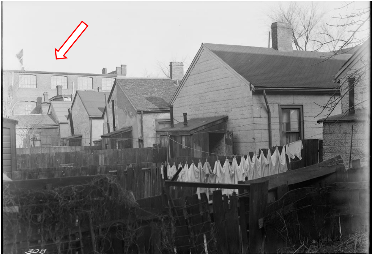
Figure 8: 1938 photograph of rear of properties along Richmond Street West; location of 822 Richmond Street West indicated by the arrow.
