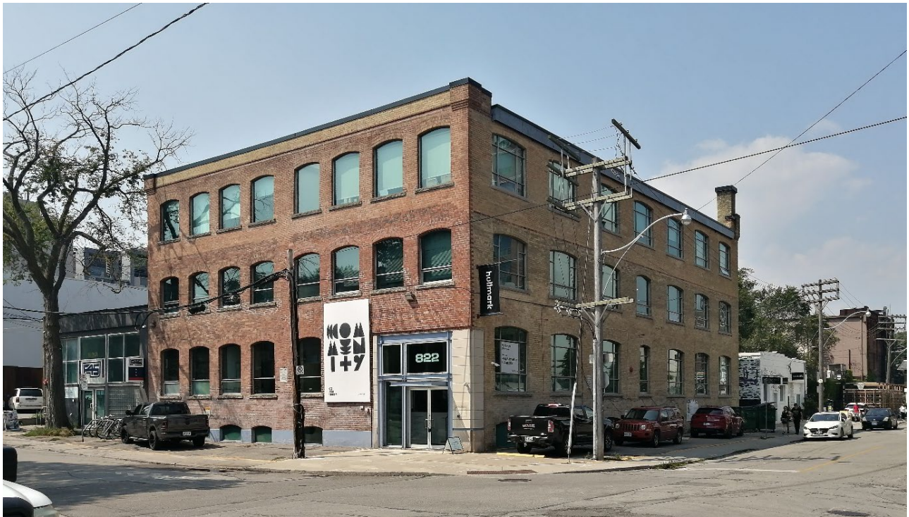
Figure 1: 822 Richmond Street West (Heritage Planning, 2023).
