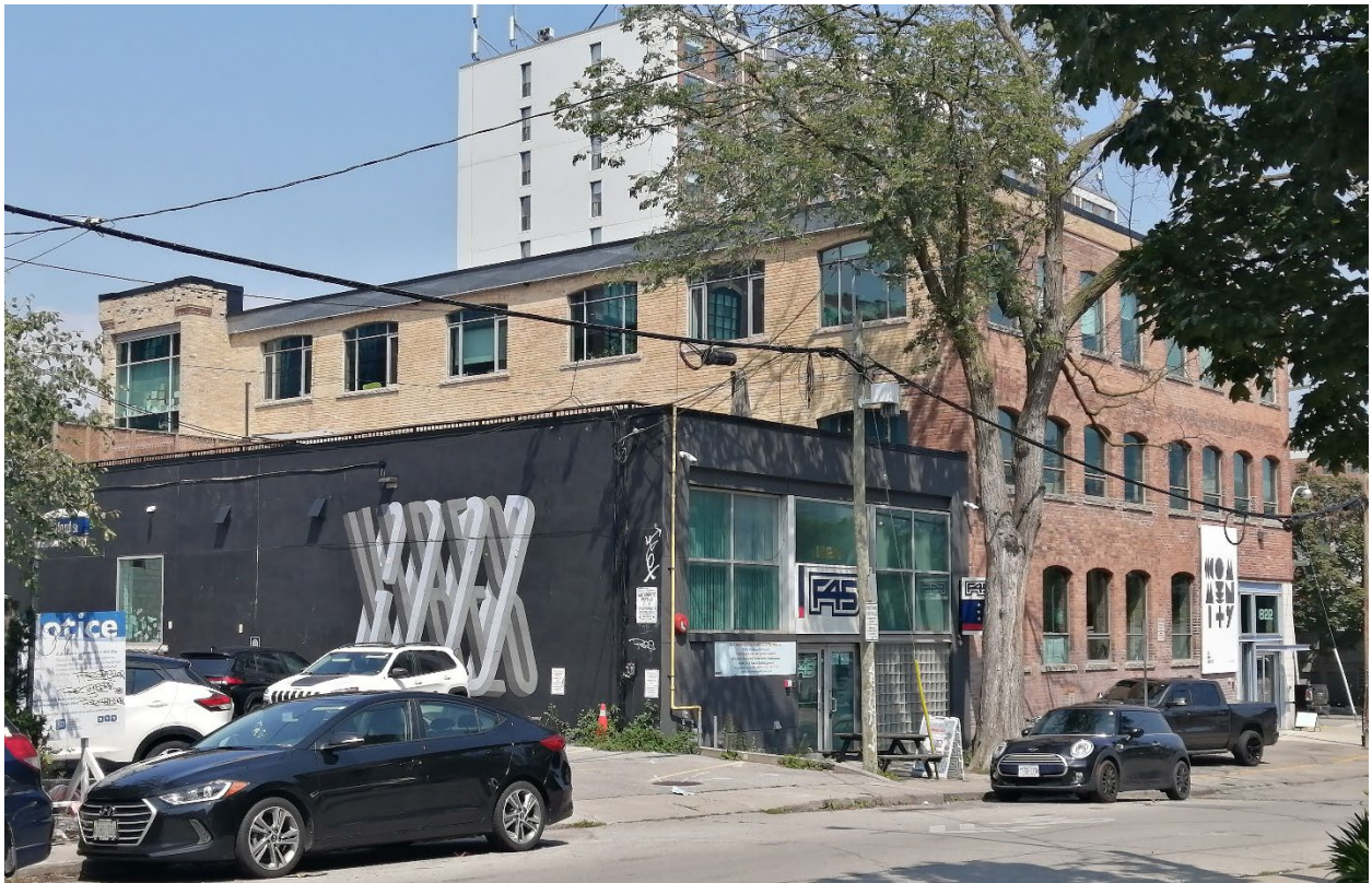
Figure 15: West and south elevations of 822 Richmond Street West viewed from Richmond Street West with 828 Richmond Street to the left (Heritage Planning, 2023).
