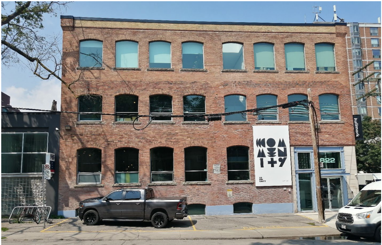
Figure 13: Primary (south) elevation of 822 Richmond Street West. (Heritage Planning, 2023).
