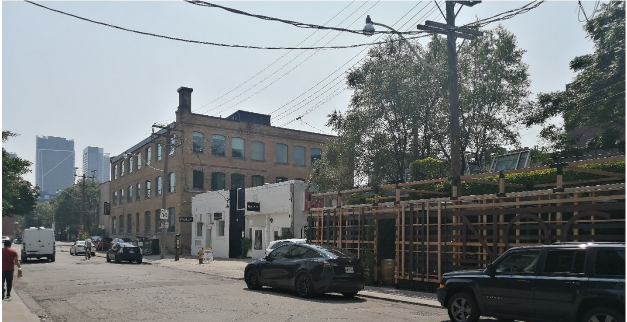
Figure 16: West and south elevations of 822 Richmond Street West viewed from Walnut Avenue (Heritage Planning, 2023).
