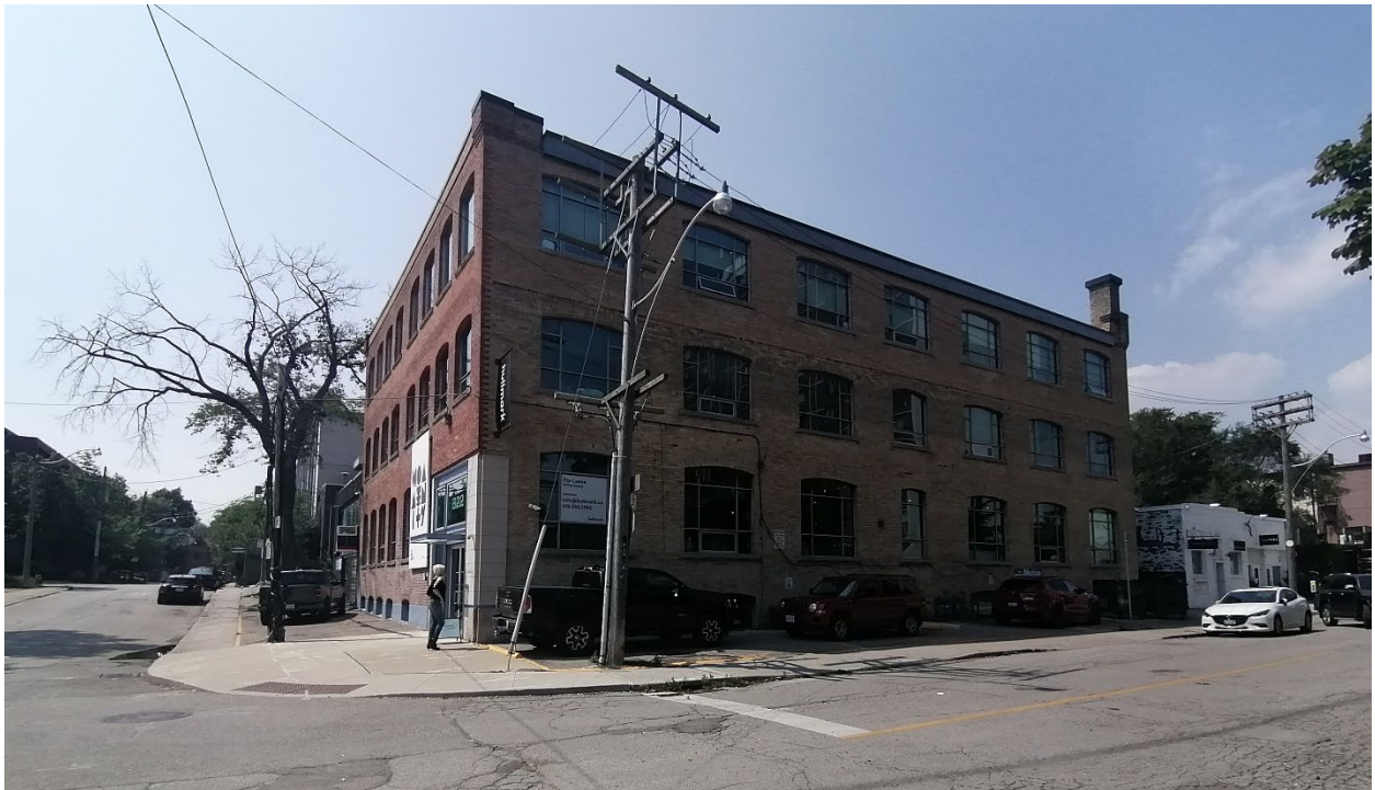
Figure 21: Northwestward view of 822 Richmond Street West from Walnut Avenue; 850 Richmond Street West to the left (Heritage Planning, 2023).
