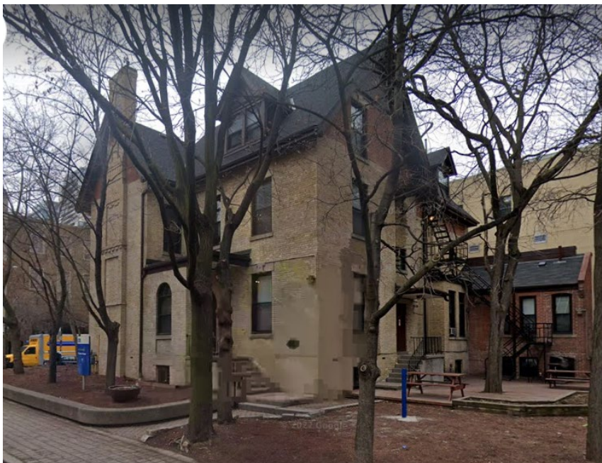
West (Bond St) elevation and south elevation
