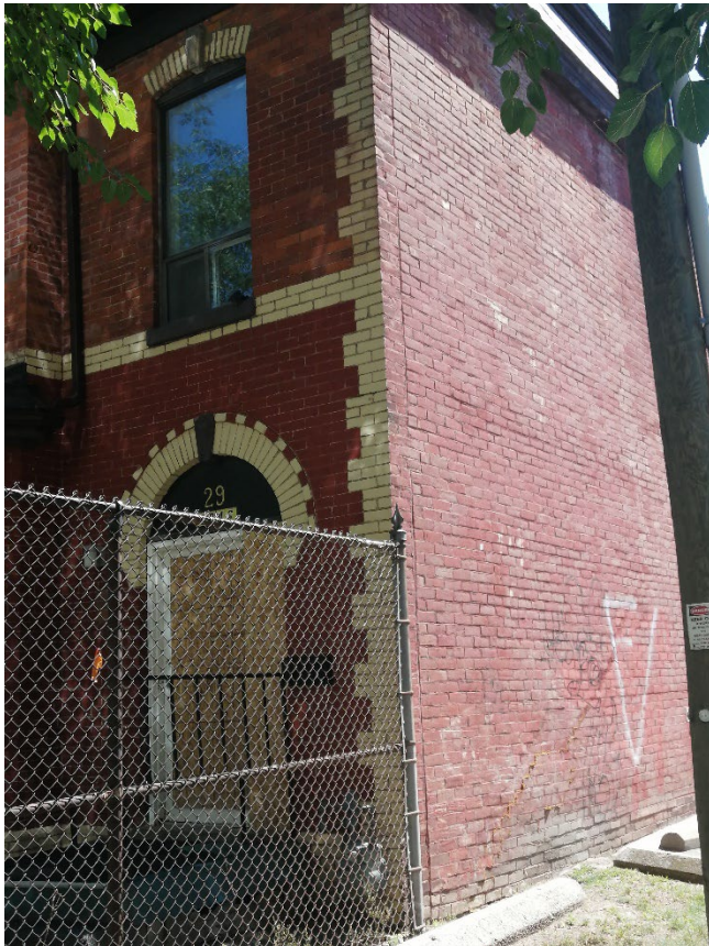
Figure 22 Northwest corner of 29 Linden Street. Note running masonry joint from later addition of brick cladding to the west elevation (Heritage Planning, 2023).
