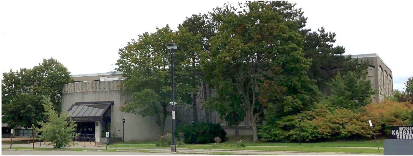
Main (north) façade of 55 Yeomans Road, Heritage Planning, 2023.
