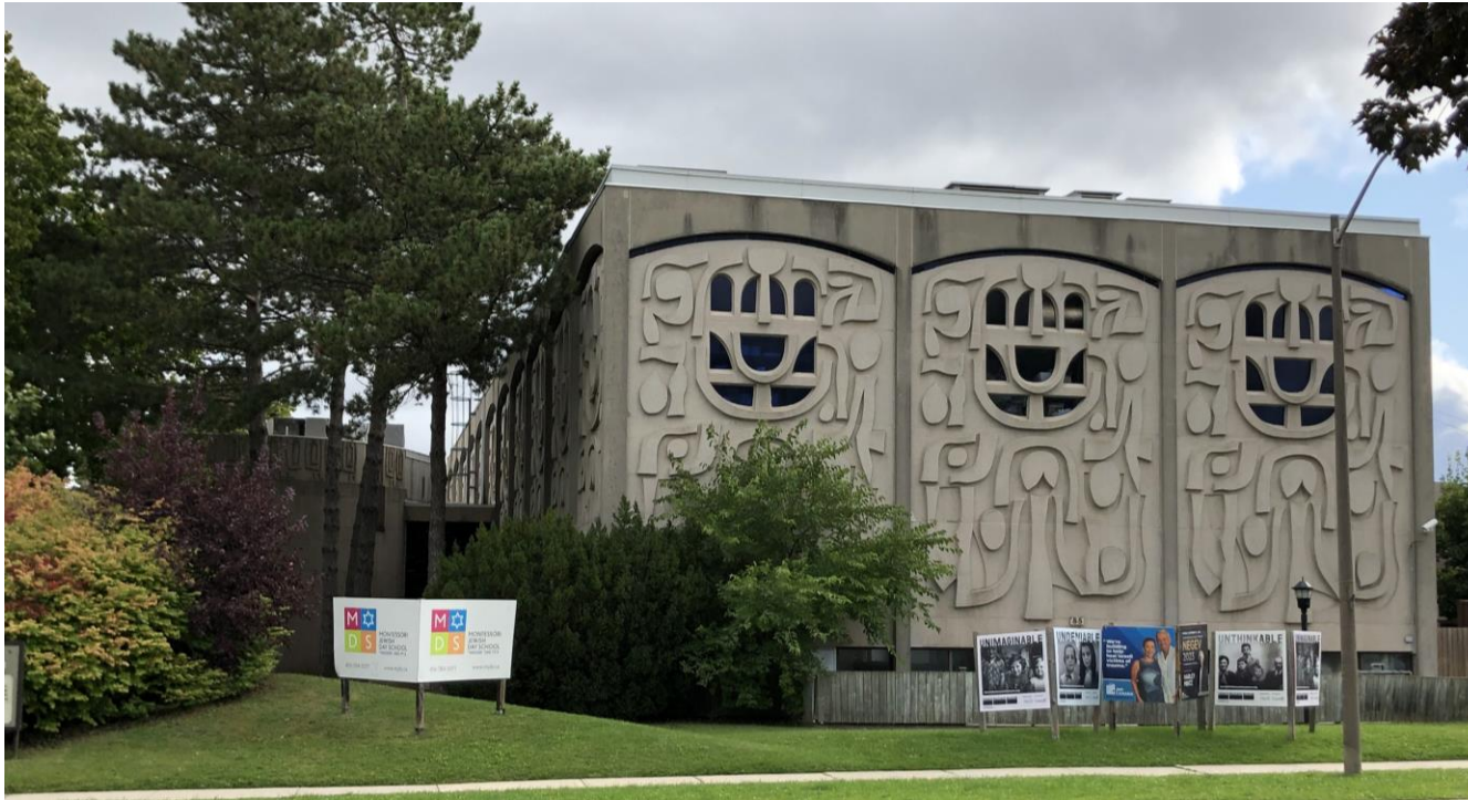
View of north (partial) and west façades. Heritage Planning, 2023.
