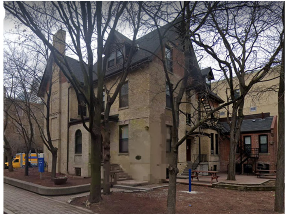
West (Bond St) and south (rear) elevations
