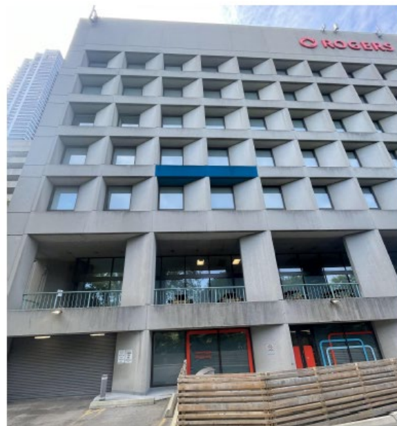
North Elevation – Site Photo
