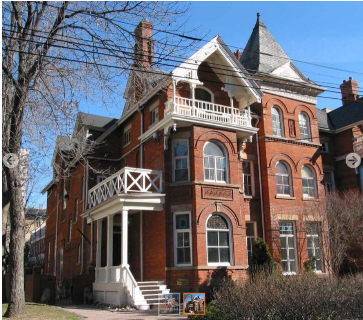
90A Isabella Street (left) Source: Bob Krawczyk/Architectural Conservancy of Ontario
