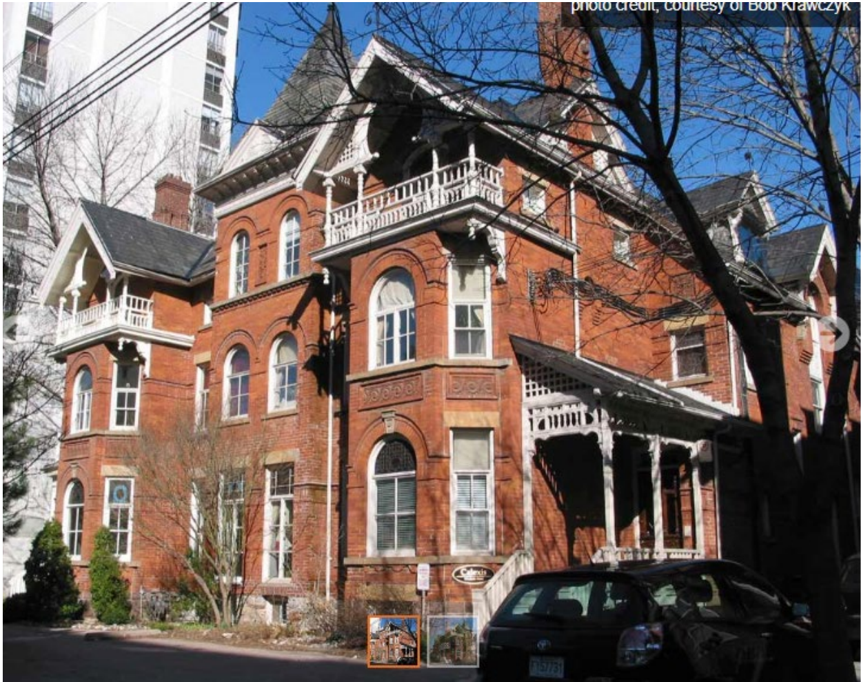
92 Isabella Street (right) Source: Bob Krawczyk/Architectural Conservancy of Ontario
