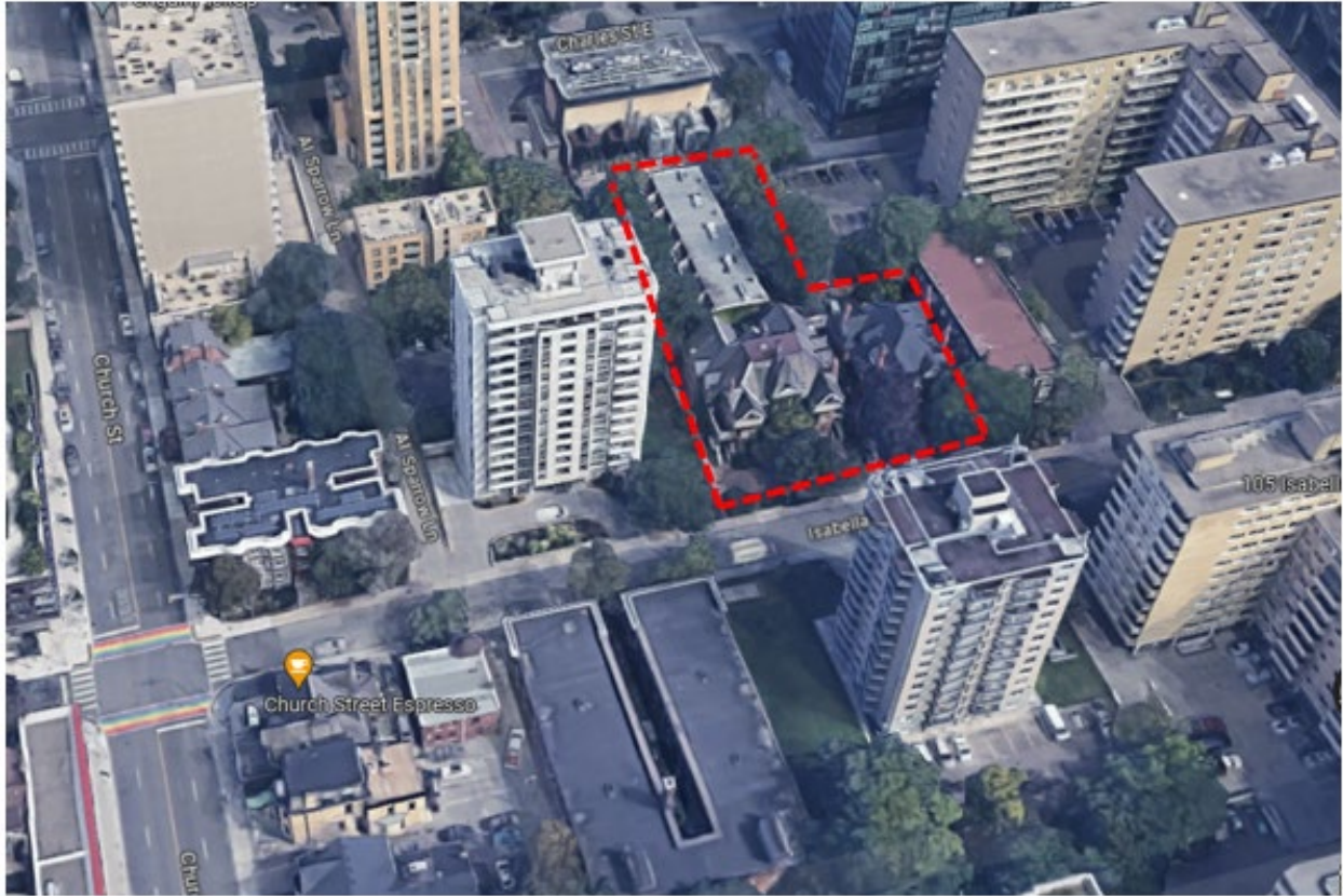
View of site looking north-east
