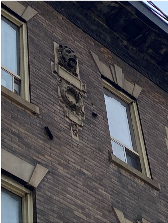
25. (left) and 26. (right) Architectural details in stone, buff-brick cladding in Don Valley brick, prominent metal cornice painted in black (Heritage Planning, 2023)
