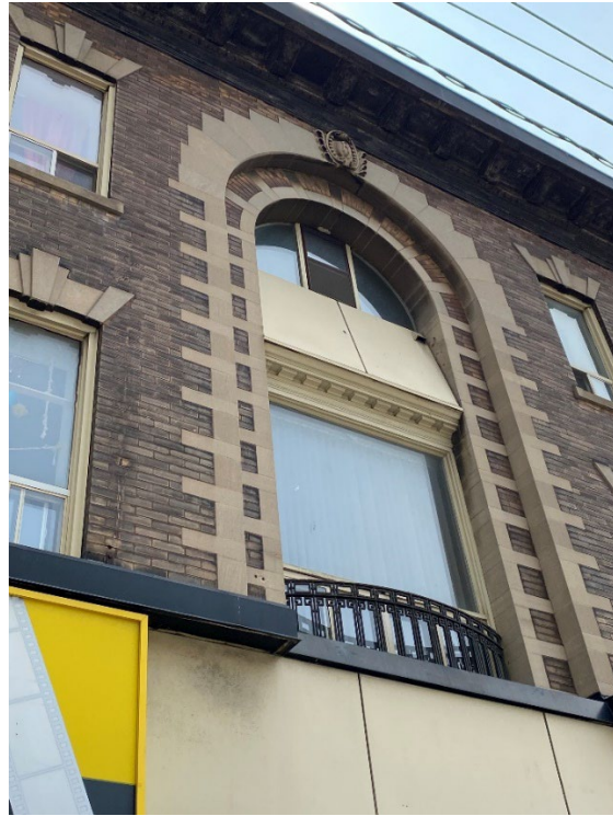
25. (left) and 26. (right) Architectural details in stone, buff-brick cladding in Don Valley brick, prominent metal cornice painted in black (Heritage Planning, 2023)
