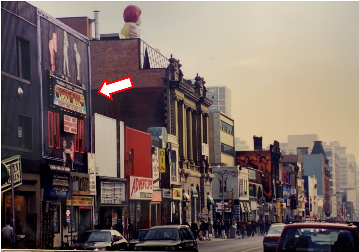
Figure 15. Archival photograph from 1991. Window openings that generally match the size and orientation of the original building can be observed on the second floor of 699 Yonge Street, outlined in neon lighting. The steel cladding on 707 Yonge Street is visible (City of Toronto Archives, Fonds 2043, Series 2573).
