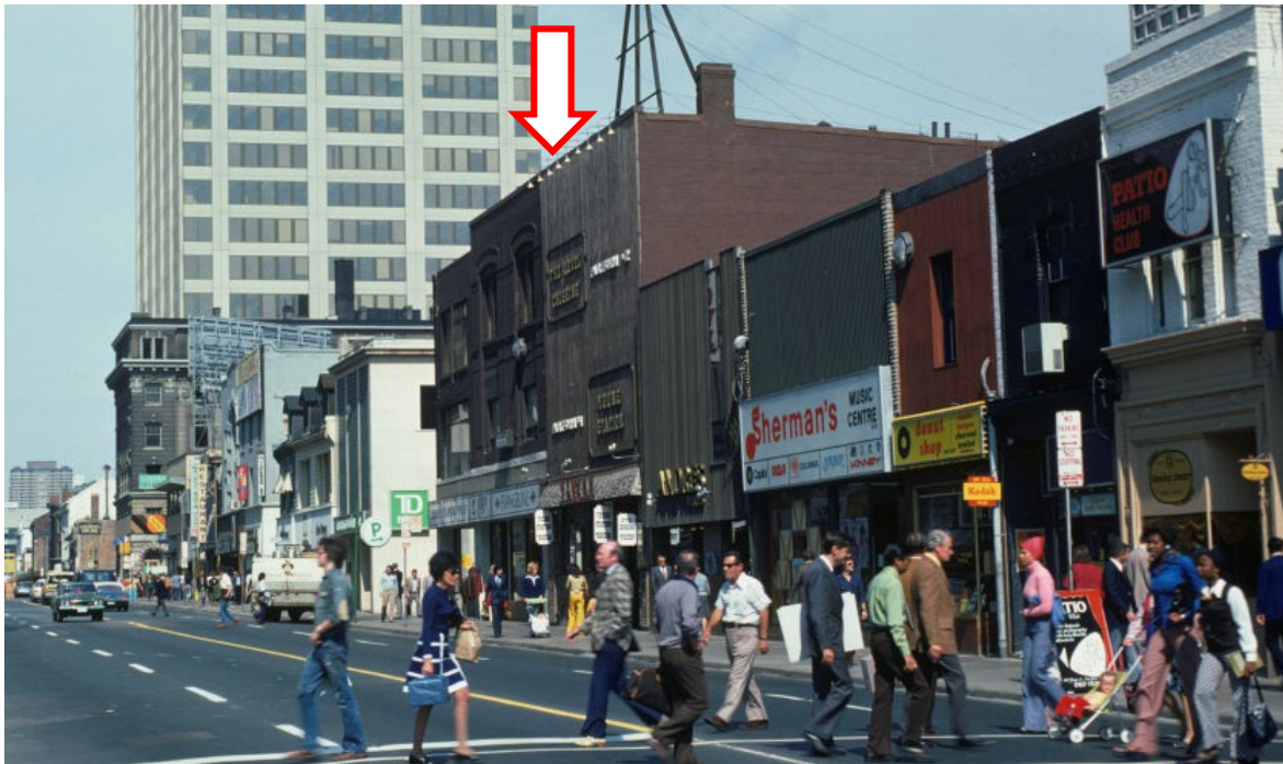
Figure 14. Archival photograph from 1974, showing the wood siding on 699 Yonge Street. The northern half of the row building (entrances at 703-705 Yonge Street) has not yet been over-clad (City of Toronto Archives, Fonds 1526, File 2, Item 8).
