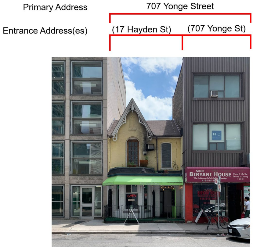
Figure 6. Partial north elevation 707 Yonge Street, with entrance addresses indicated. (Heritage Planning 2023).
