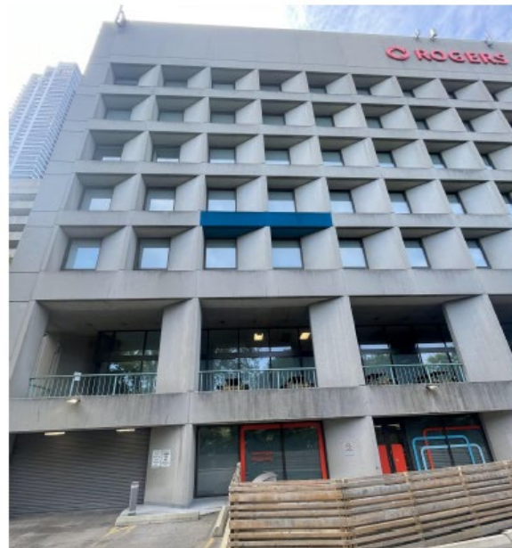
North Elevation – Site Photo
