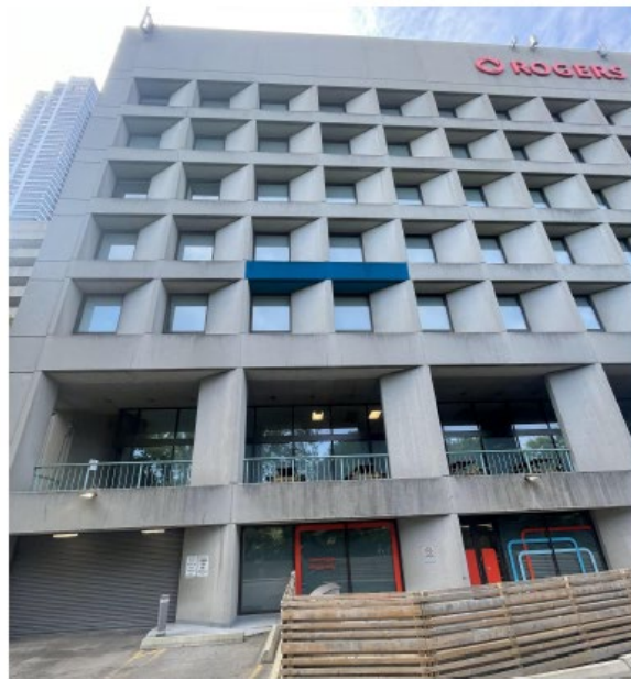
North Elevation – Site Photo
