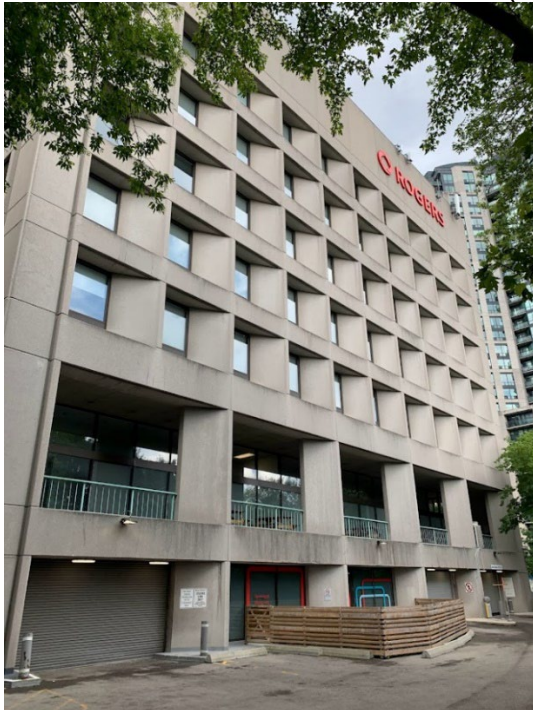
View showing the north elevation with the colonnaded pedestrian terrace and exposed lower level containing the entrance to the second lower level parking garage. (Heritage Planning, 2023)
