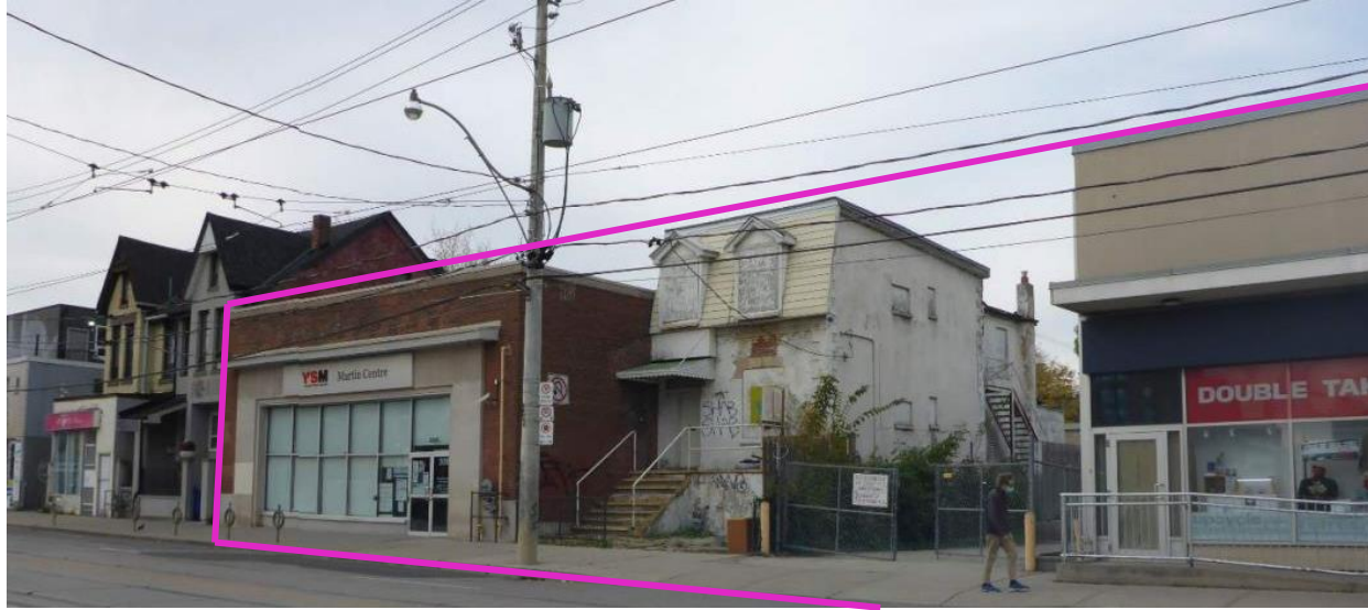
Existing buildings at 306 & 308 Gerrard Street East. (Design Workshop Architects, 2021)
