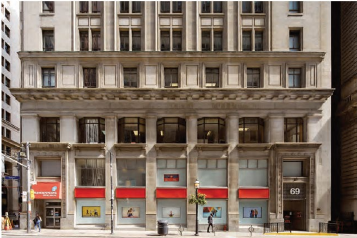
View of the Yonge Street (west) elevation plinth
