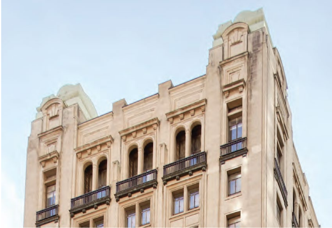
View of the crown facing King Street East
