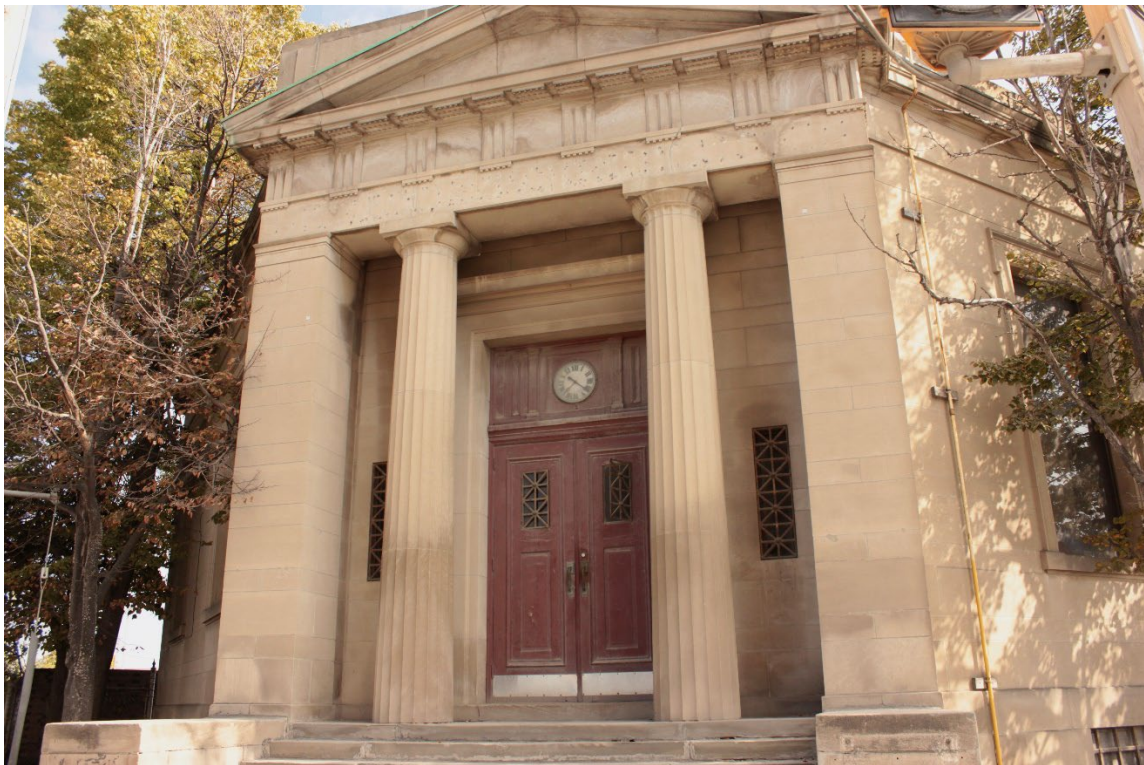
Figure 16. Main entrance details (Heritage Planning, 2023).
