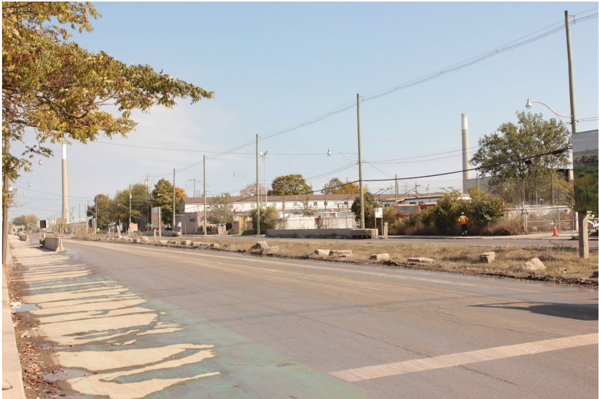
Figure 41. Looking east down Villiers Street (Heritage Planning, 2023).
