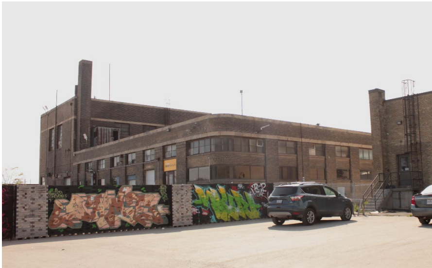
Figure 29. Northeast elevation (Heritage Planning, 2023).
