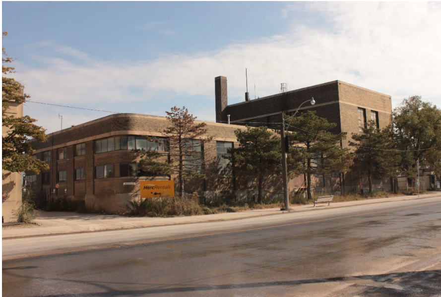
Figure 28. Northwest elevation of former Canadian Oil Companies warehouse (Heritage Planning, 2023).
