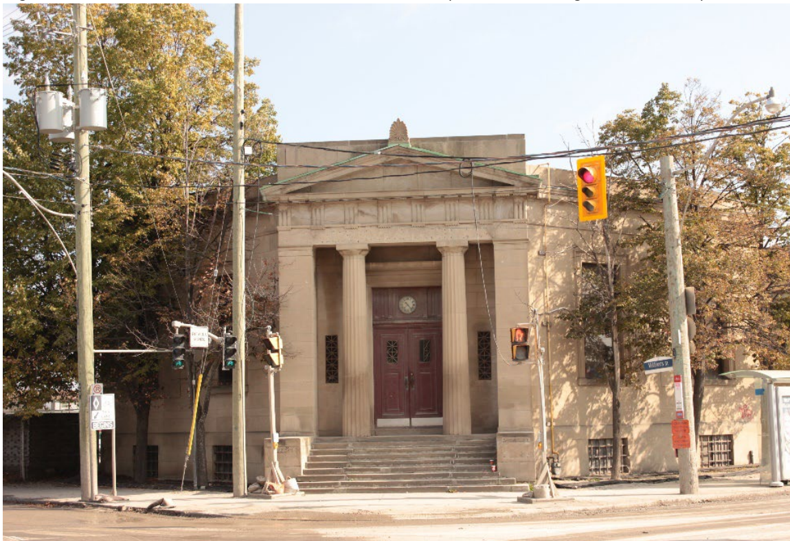
Figure 14. Northwest corner of former Bank of Montreal (Heritage Planning, 2023).
