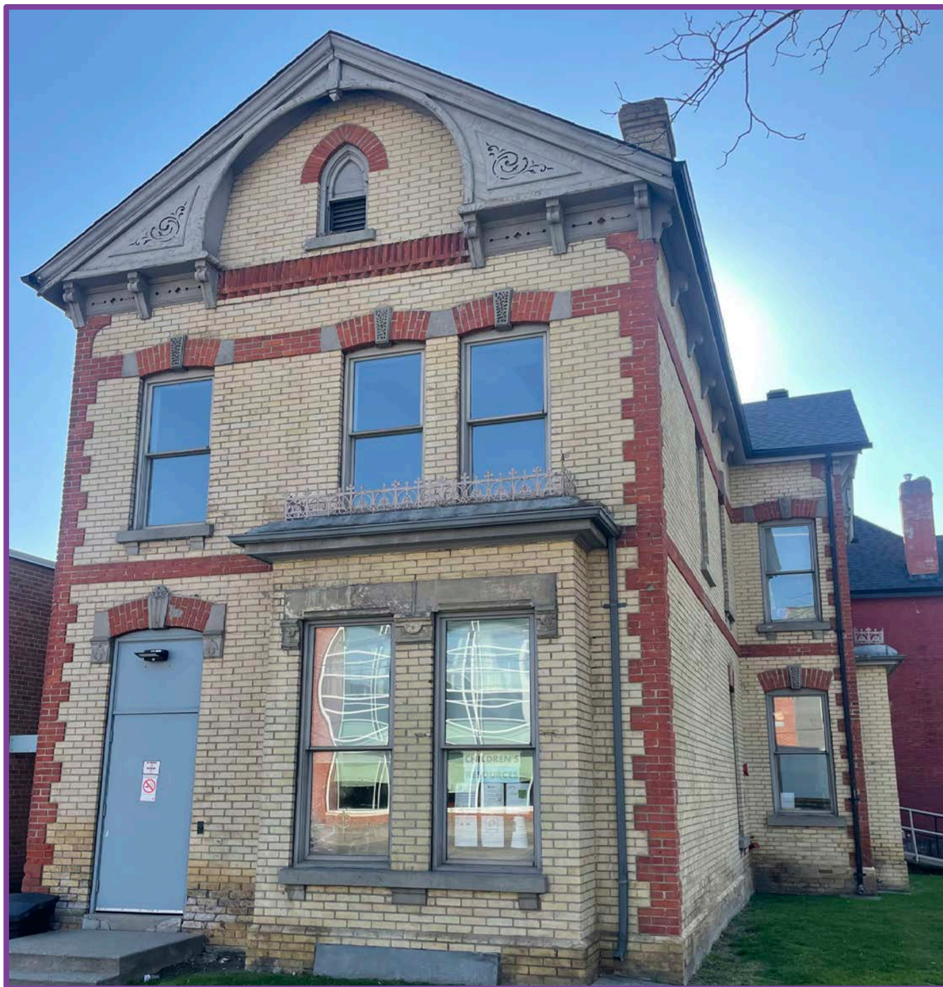
Figure 50: Toronto Public Library - 265 Gerrard St. E.
