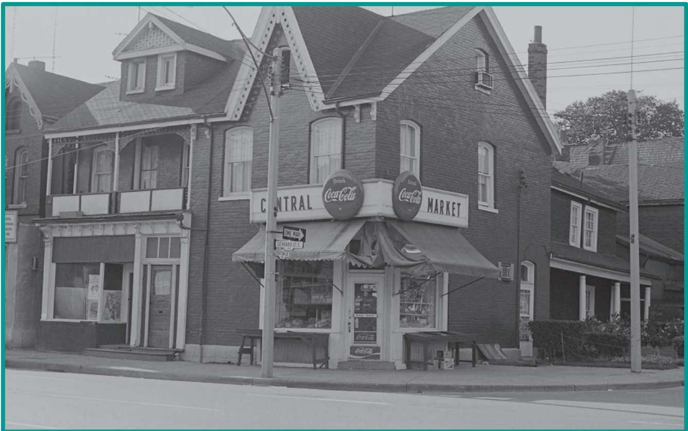
Figure 14: Corner of Seaton St. and Gerrard St. E, looking northwest, c. 1972, City of Toronto Archives.
