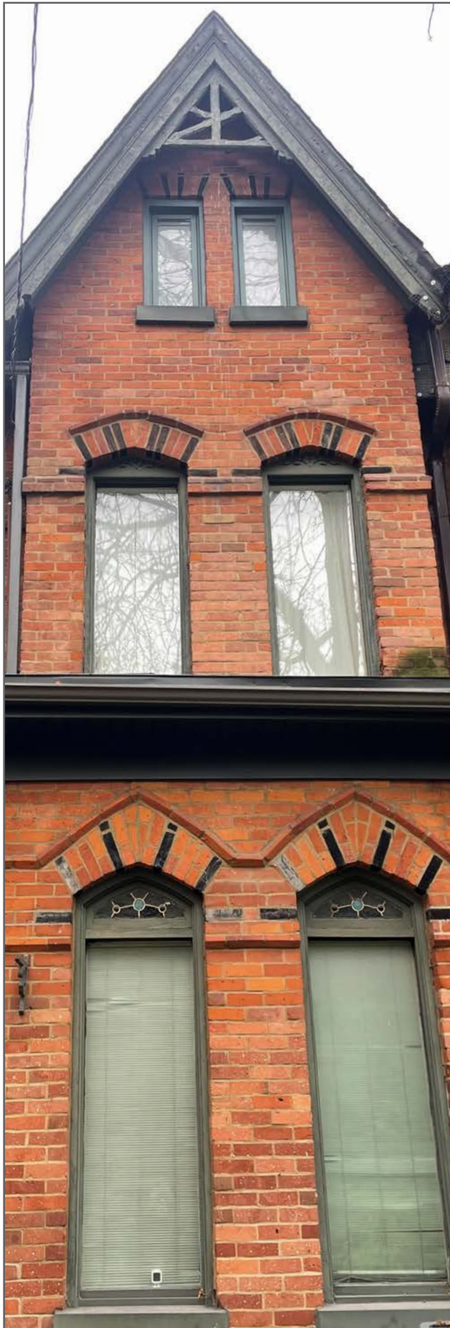
Figure 68: Retention of ground floor transom lights at 175 Seaton St.
