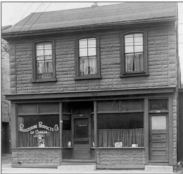
Figure 80: Demolished property at 168 Ontario St., 1951, City of Toronto Archives.
