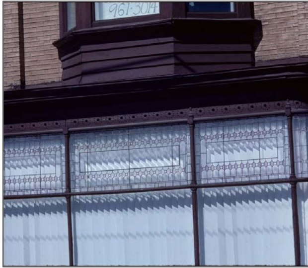
Figure 71: Historic storefront details at 412 Dundas St. E., 1984, City of Toronto Archives.
