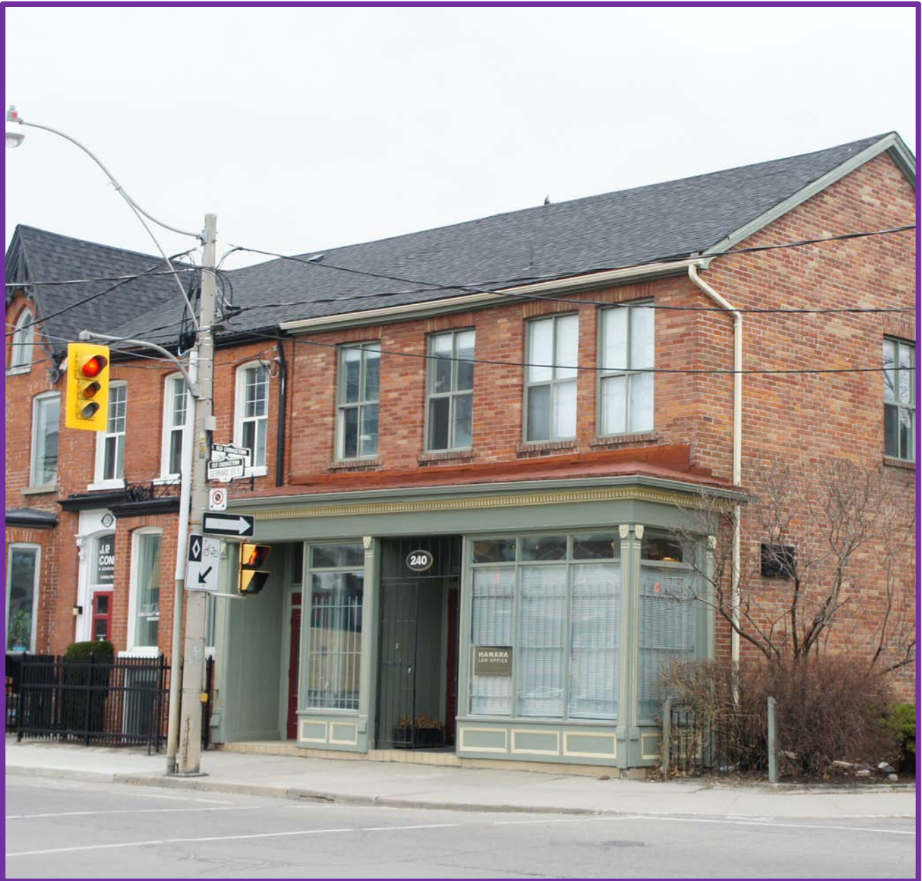
Figure 70: Historic storefront at 240 Gerrard St. E.
