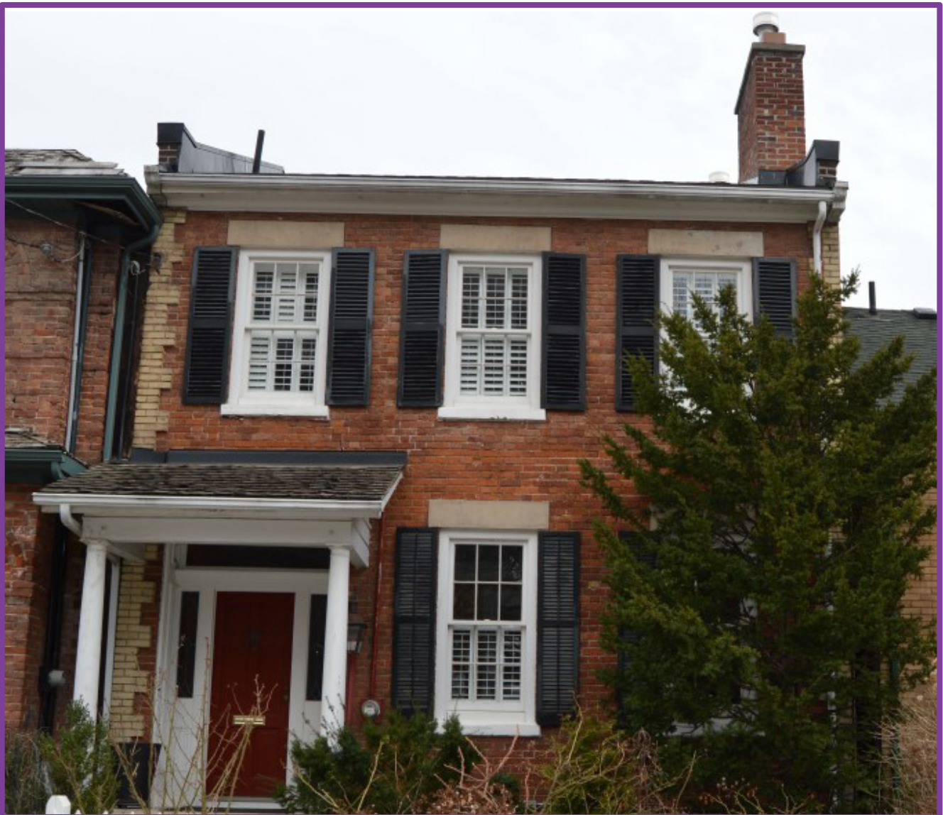
Figure 52: An example of a Part IV designated property at 77 Seaton St.
