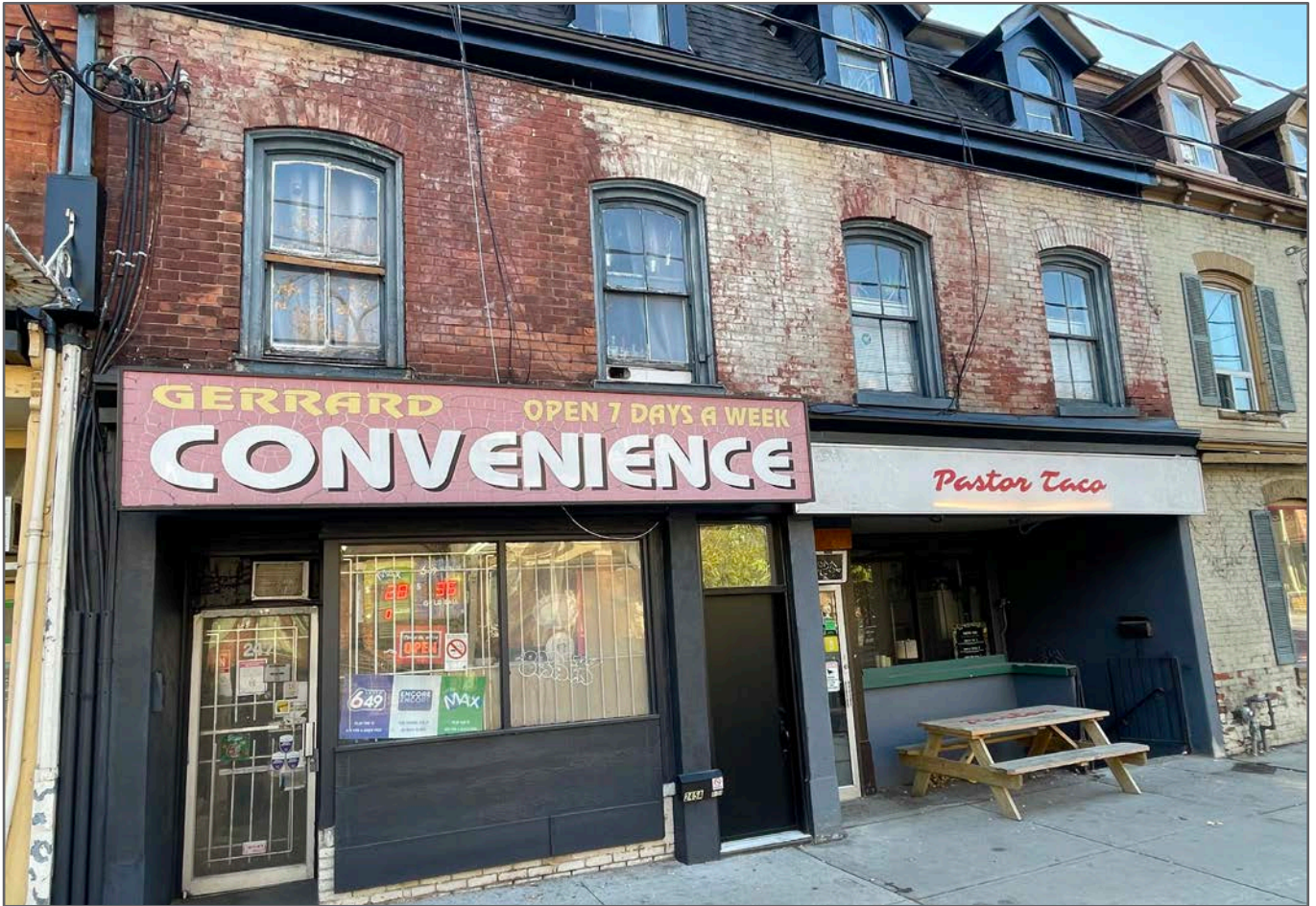
Figure 72: Gerrard St. E. storefront with non-historic finishes.
