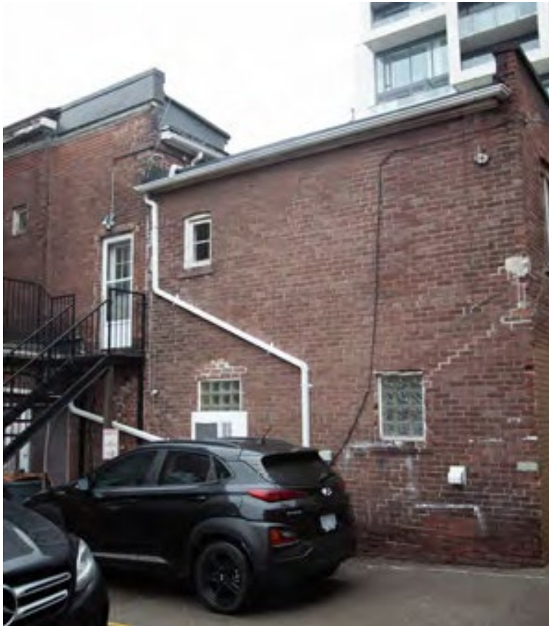
Figure 12 2111 Yonge Street south elevation (ERA Architects Inc, 2023).
