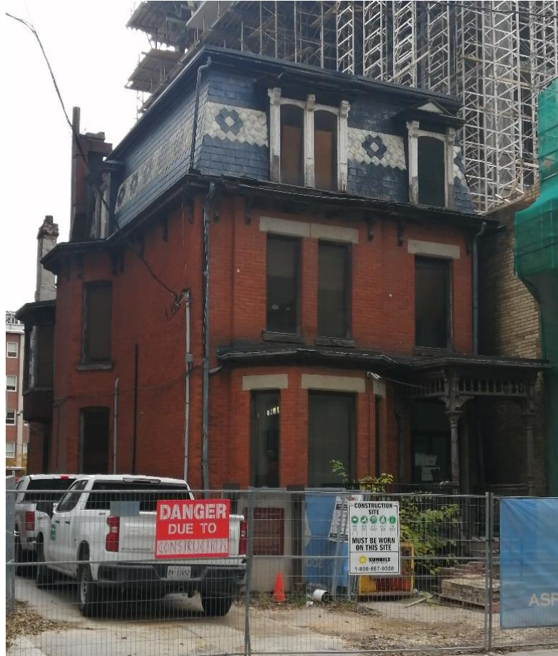
South and west elevations of 66 Charles Street East (Heritage Planning, 2023).
