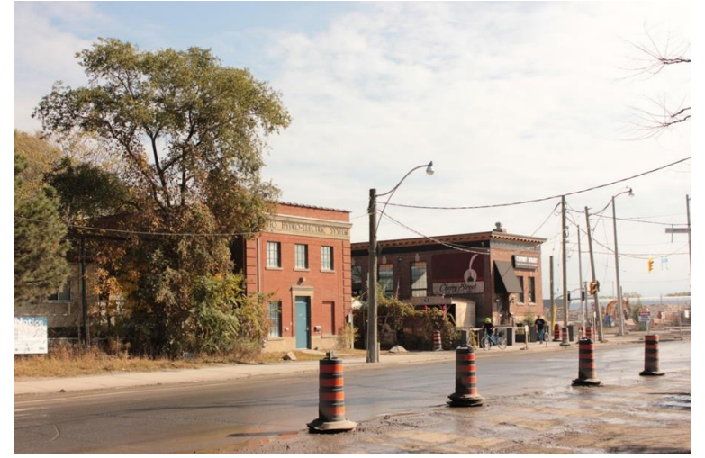
Toronto Hydro Substation and former Dominion Bank at Cherry and Commissioners streets.
