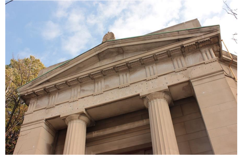
Detail of main entrance portico pediment and entablature (Heritage Planning, 2023).
