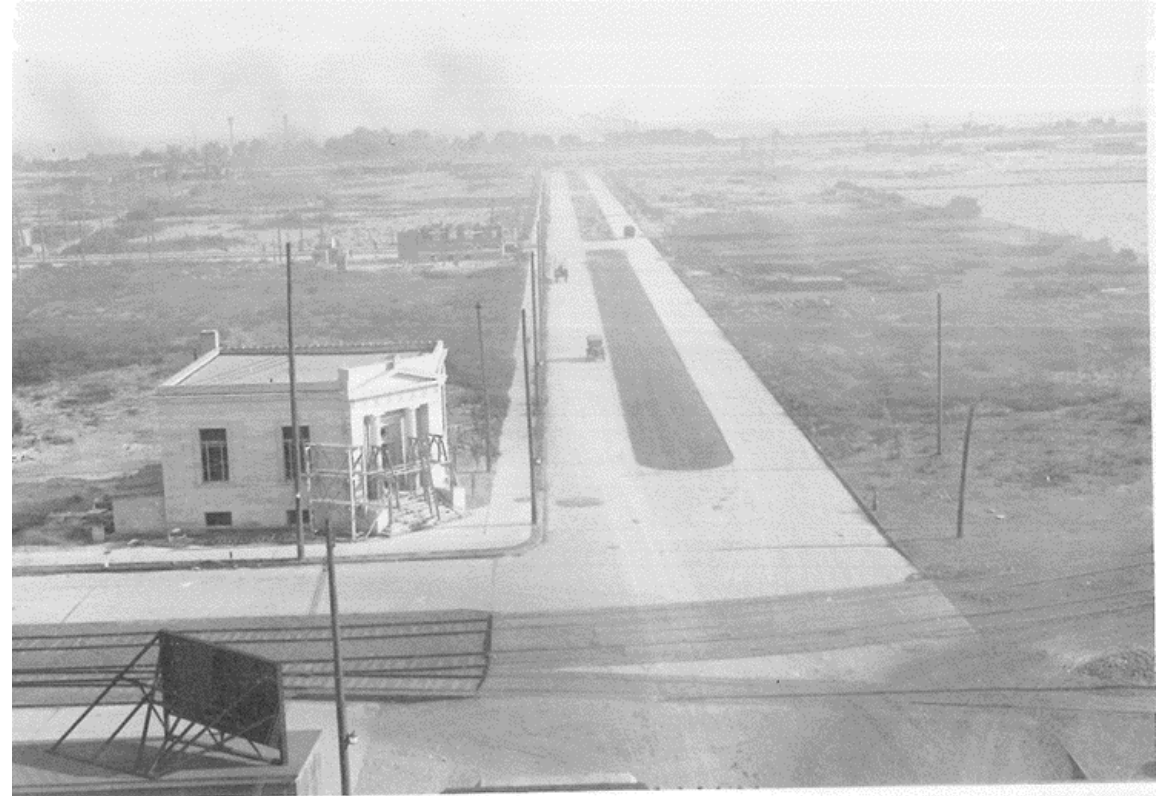
Bank of Montreal under construction in 1920, from "Heritage Impact Assessment: 309 Cherry Street, Toronto." ERA Architects, Inc. 2023.
