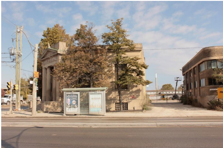
Former Bank of Montreal's west elevation, looking east and showing space between buildings.
