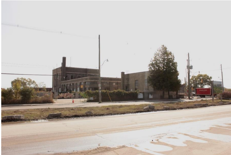
East elevations of buildings looking southwest.
