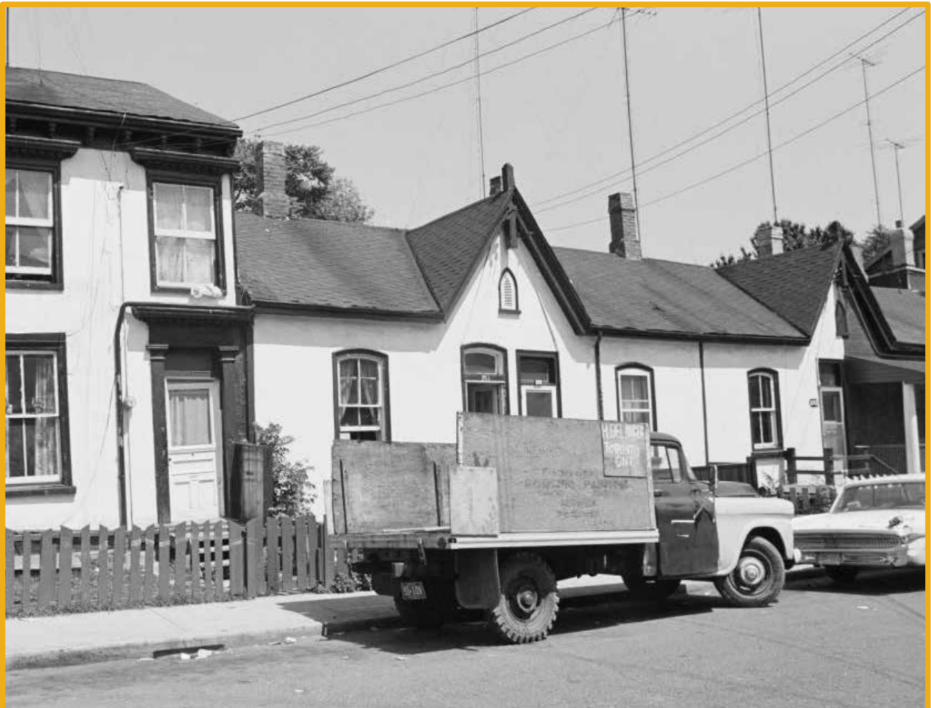
Figure 10: East side of Ontario St., south of Dundas St. E., 1972, City of Toronto Archives.
