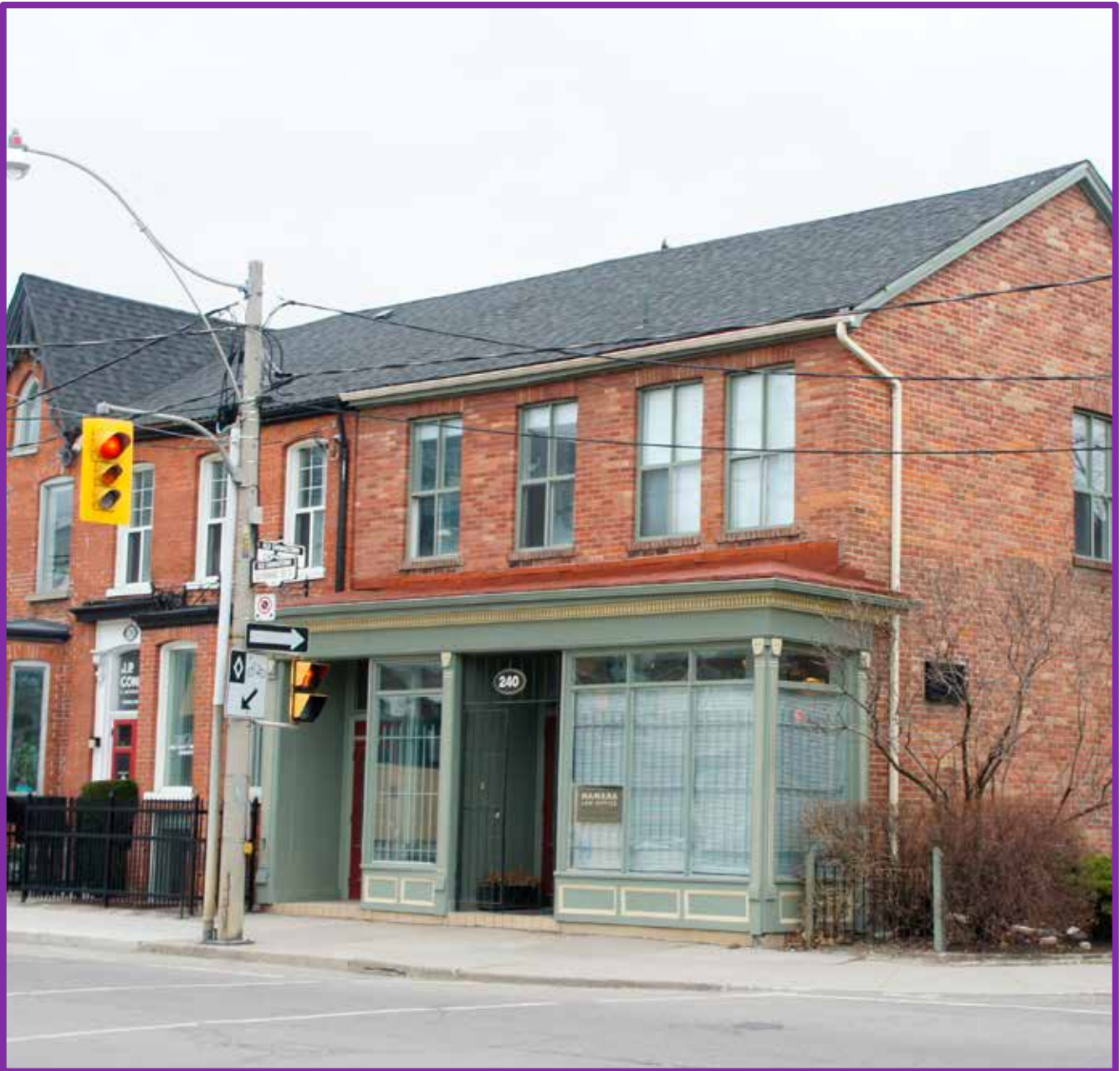
Figure 70: Historic storefront at 240 Gerrard St. E.
