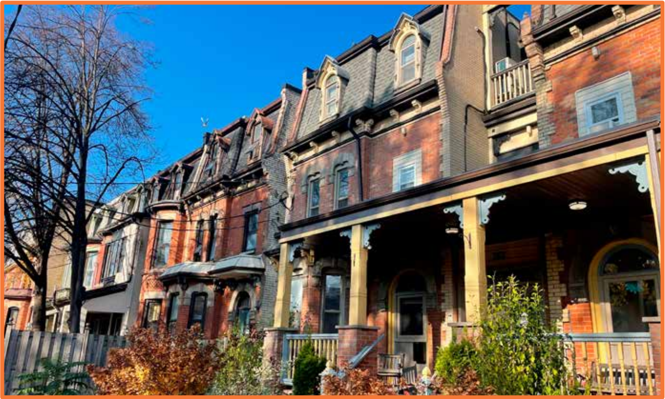
Figure 43: North side of Gerrard St. E between Berkeley St. and Ontario St.
