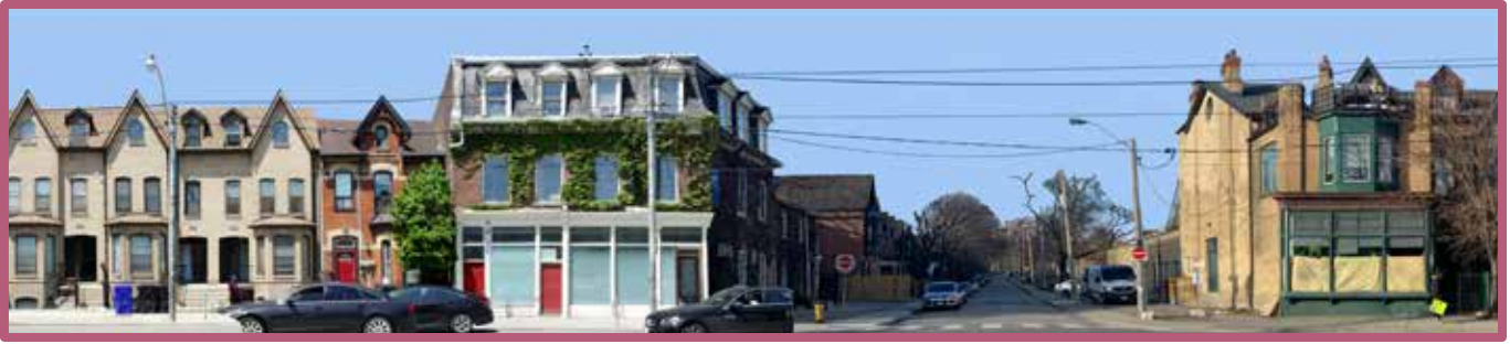
Figure 23: North side of Dundas St. E. at Berkeley St.
