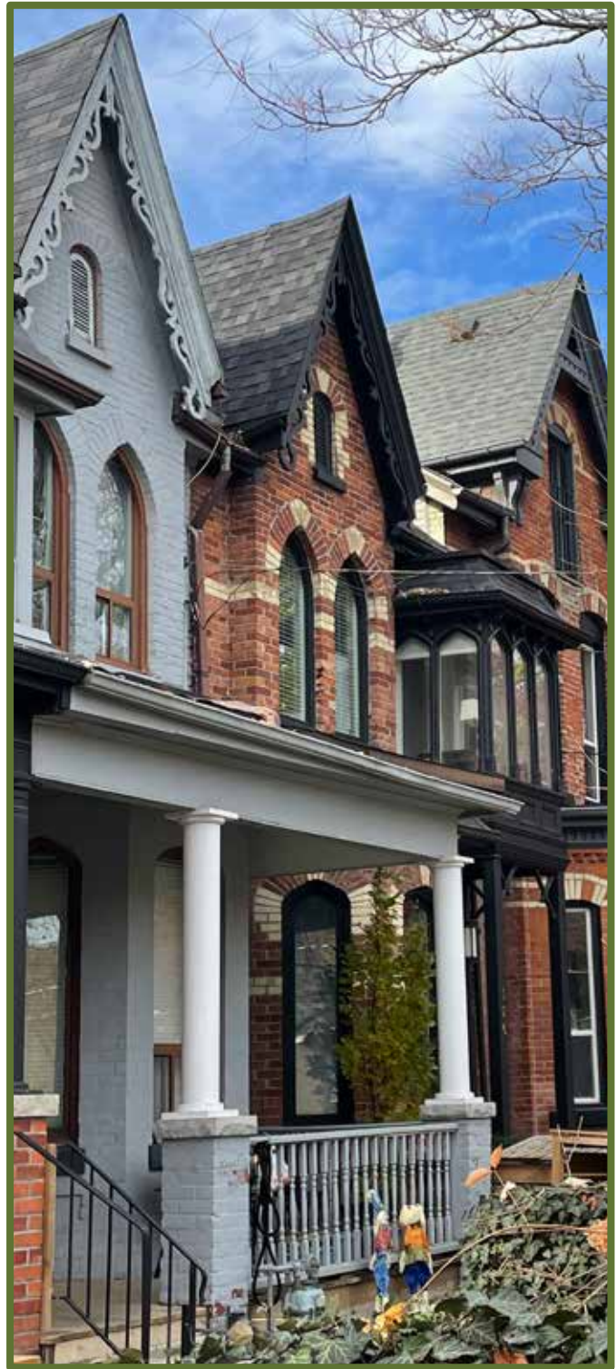
Figure 101: West side of Berkeley St north of Dundas St. E.
