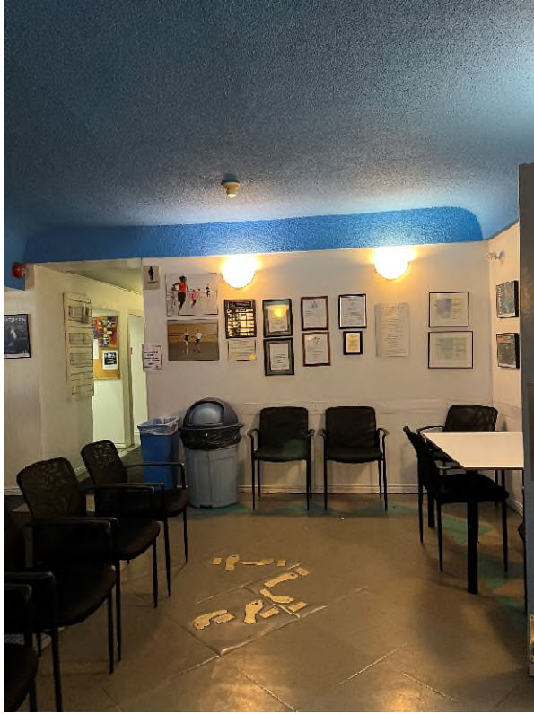
Interior of lobby (ERA, 2022).
