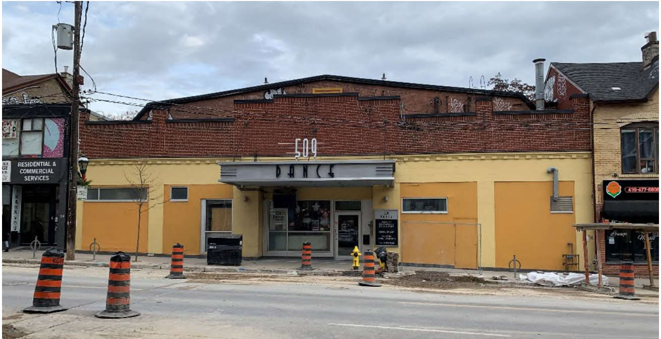
Front (west) elevation (ERA, 2022).
