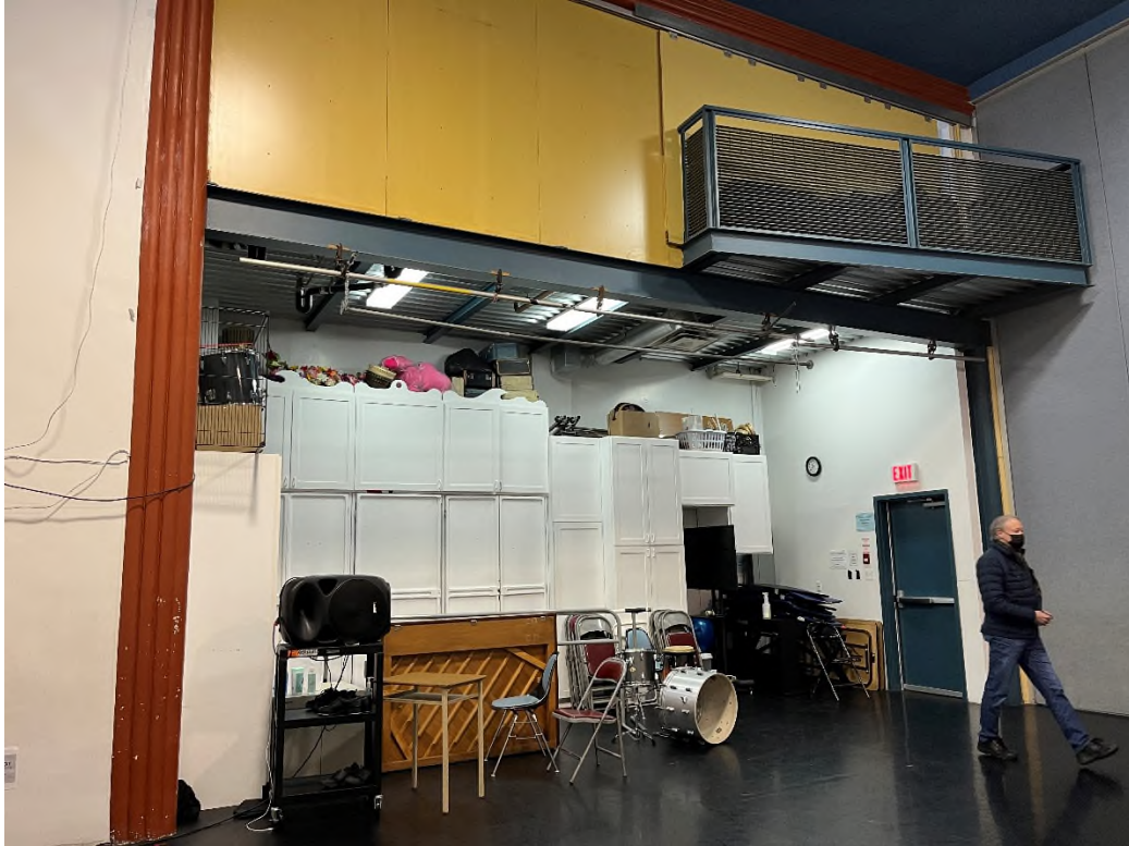
Remaining screen opening mouldings (ERA, 2022).
