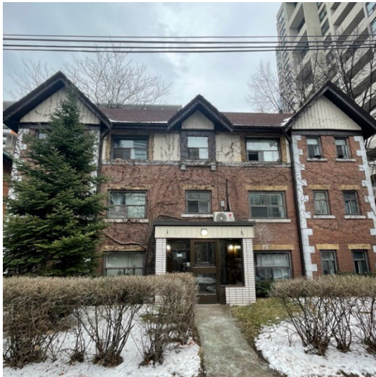
33 Maitland Street, Heritage Planning 2022.
