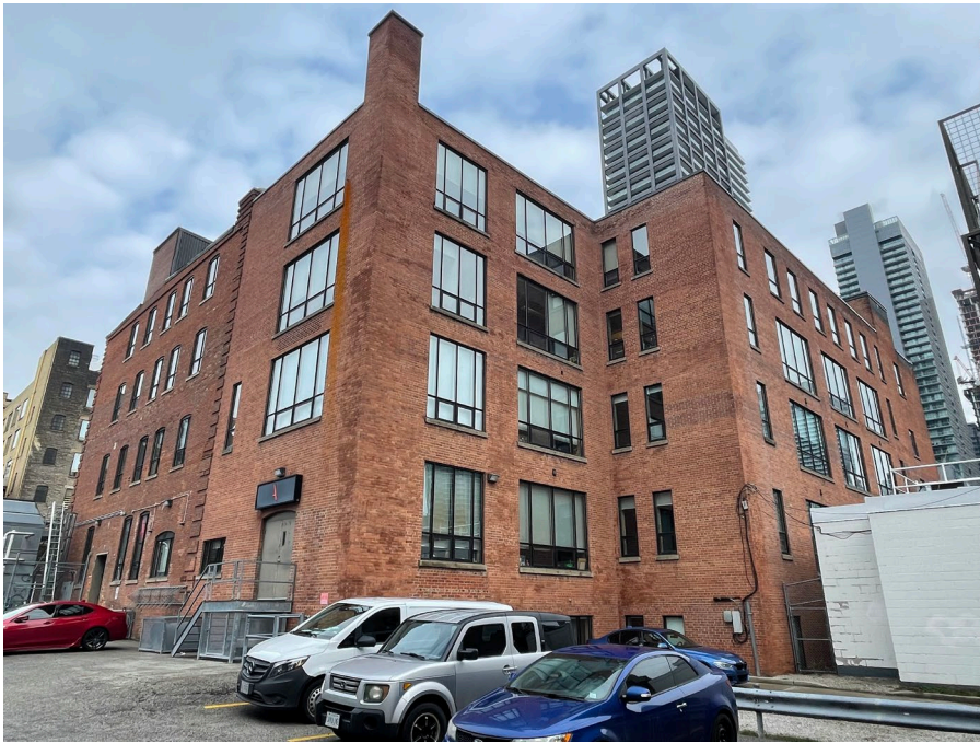
Figure 10: Southwest corner of the property at 46 Spadina Avenue, 2022. (Heritage Planning)
