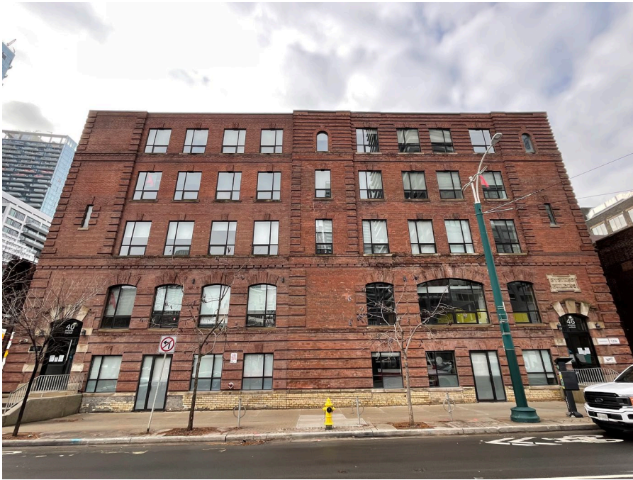
Figure 8: East (principal) elevation of the property at 46 Spadina Avenue, 2022. (Heritage Planning)
