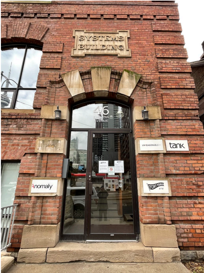
Figure 13: Detail of the primary entry on the west elevation of the subject property, 2022. Note Gibbs surround and Systems Building name plate. (Heritage Planning)
