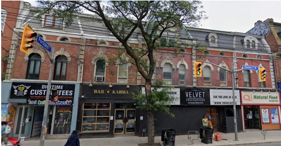
Figure 8: 506-514 Queen Street West - designed by William Stewart in 1874; a contributing property of the Queen Street West Heritage Conservation District.
