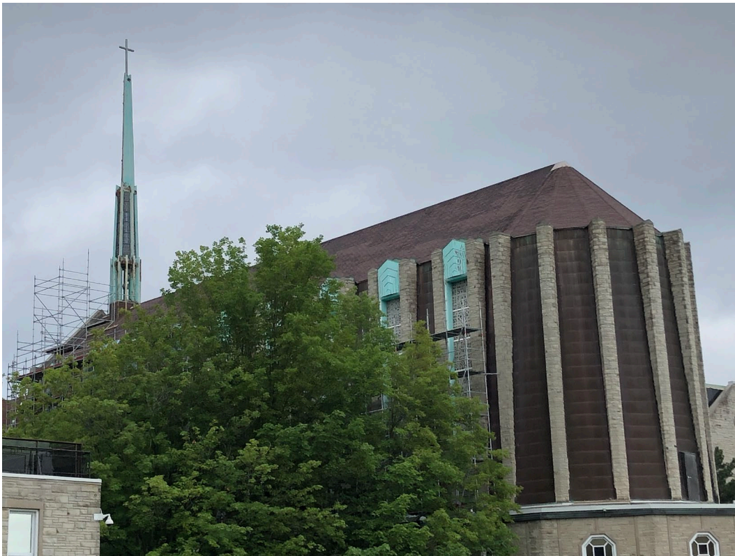
Figure 16: Exterior view of the Motherhouse Chapel and steeple, 2021 (Heritage Planning).
