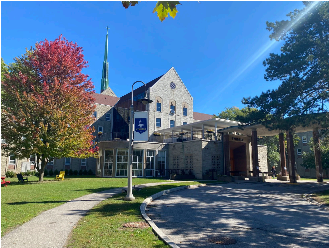
Figure 13: Primary entry and porte-cochère to the Motherhouse building, 2022 (Heritage Planning).
