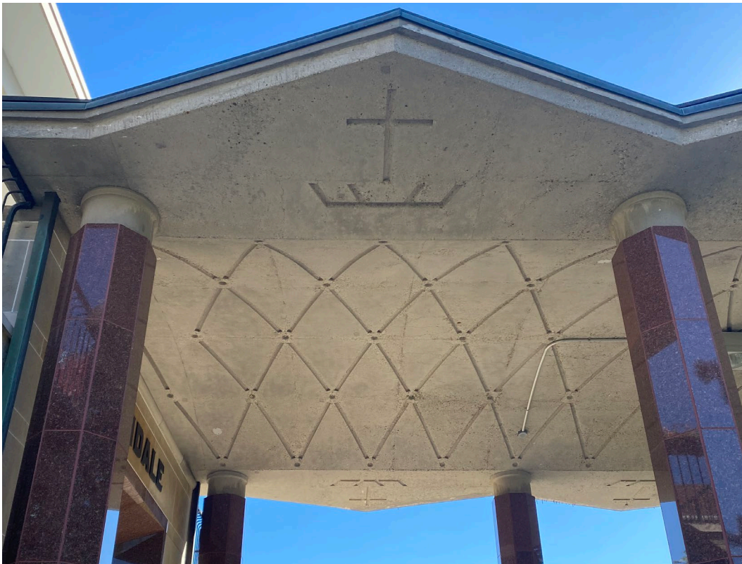
Figure 12: Details of the porte-cochère at the primary entry, 2022 (Heritage Planning).
