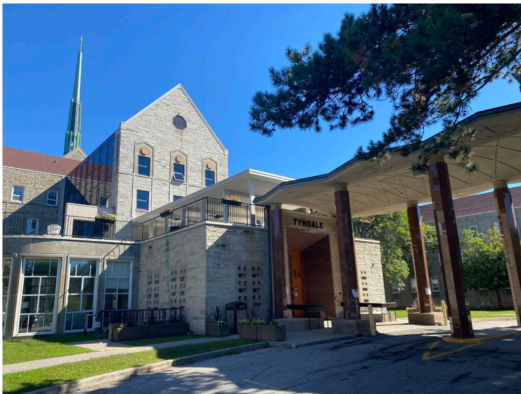
Figure 1: 3377 Bayview Avenue, primary entry to Motherhouse, 2022 (Heritage Planning).
