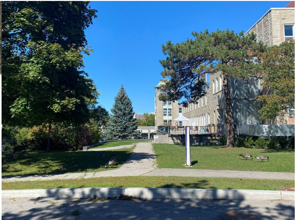
Figure 22: The view from the curve in the original circular driveway that leads from Bayview Avenue to the Motherhouse, looking north toward the Annex and school tower (Heritage Planning).
