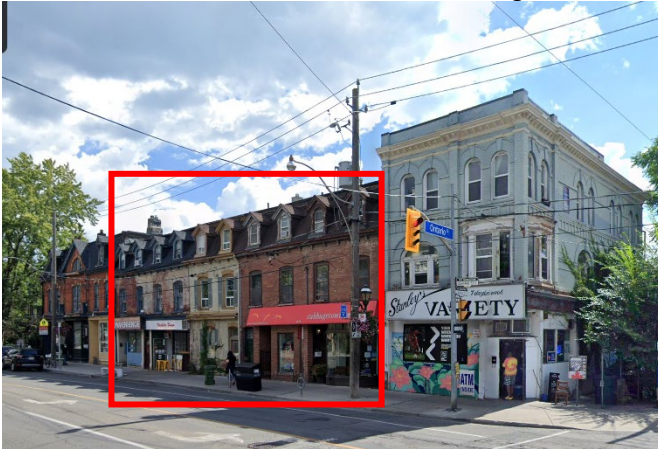
Photograph shows subject buildings (in red box) in context of 249 Gerrard Street East to the left (recommended for listing) and 237 Gerrard Street East to the right (listed 1995). Google Maps, 2021.
