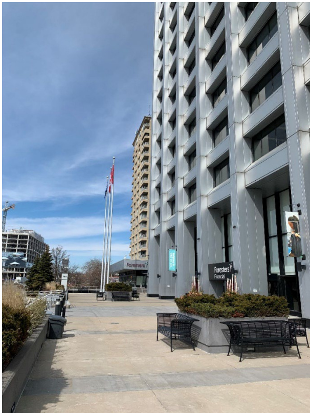
Figure 36. West side of the raised plaza, looking north, with planters and double-height first storey with piers (Heritage Planning, 2023)
