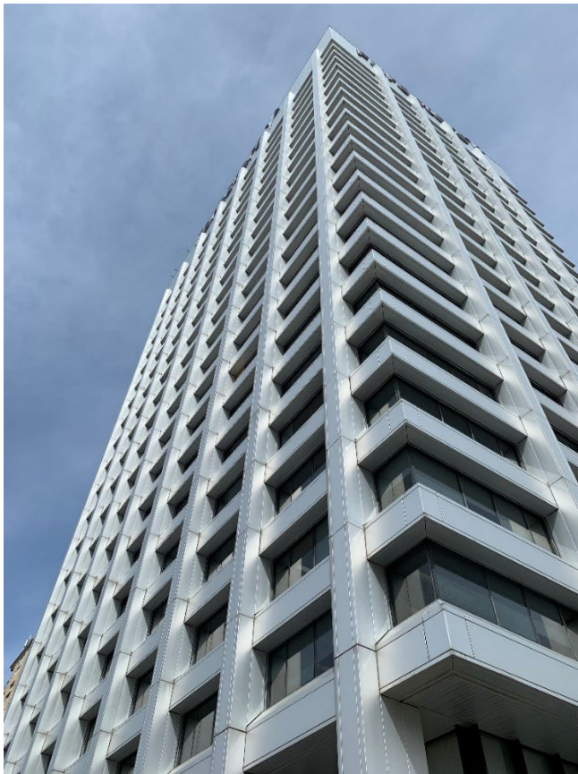
Figure 38. Southwest corner of the Foresters tower, looking northeast, showing the piers set forward from the elevation, ribbon windows, and the recessed chamfered horizontal panels beneath the windows (Heritage Planning, 2023)
