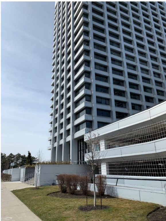
Figure 28. View of the south elevation of the Foresters tower from Rochefort Drive, looking northwest, showing the stairs leading to the raised public plaza surrounding the base of the tower building (the adjacent parking structure is not identified as a heritage attribute) (Heritage Planning, 2023)
