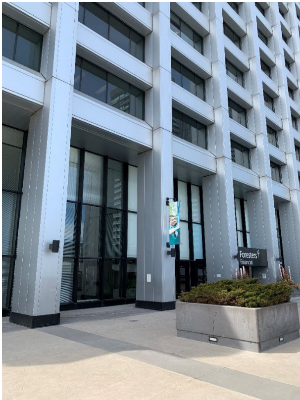
Figure 30. View of the east side of the raised public plaza, looking northwest, with planters and double-height first storey with massive piers (Heritage Planning, 2023)
