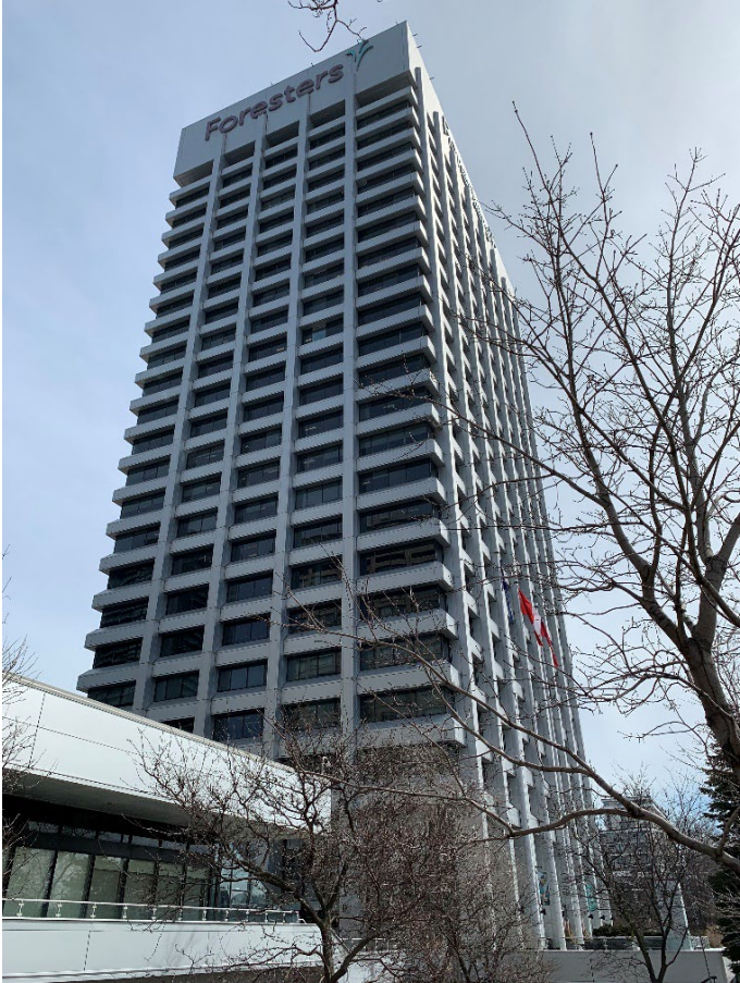
Figure 20. 789-793 Don Mills Road: north and west elevations, looking southeast (Heritage Planning, 2023)
