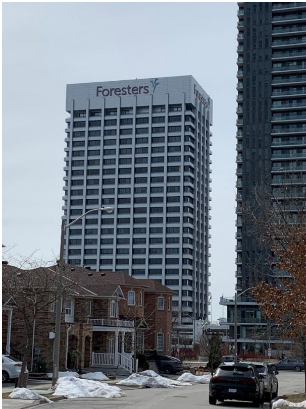
Figure 23. 789-793 Don Mills Road: east elevation viewed from Seton Park Road (Heritage Planning, 2023)
