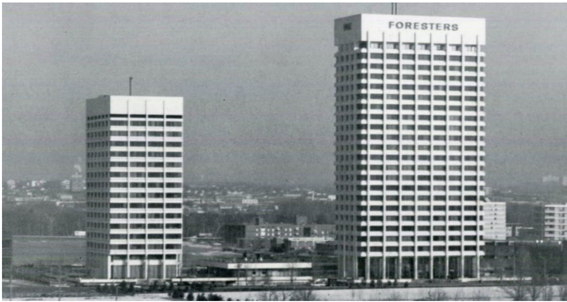
Figure 12. View of the Olympia Square, looking east, showing the two-storey pavilion on the north side of the Foresters tower (unknown photo date) 33
