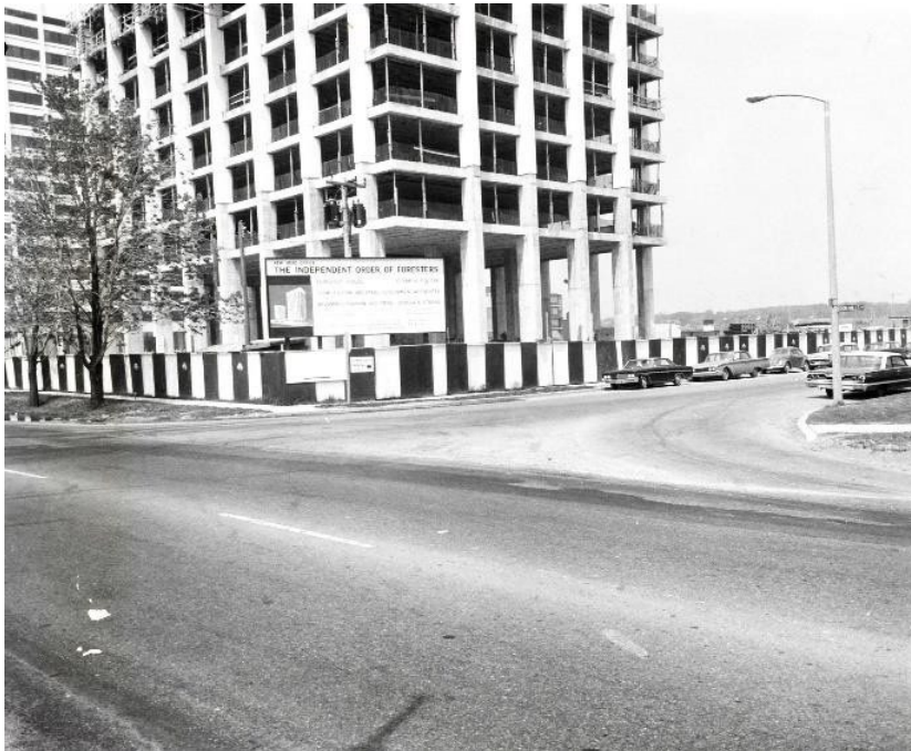
Figure 17. View northeast of the southwest corner of 797 Don Mills Road while under construction, 1966 (C.O.T.A. Fonds 220 Series 3 File 86) (ASI, 2019)
