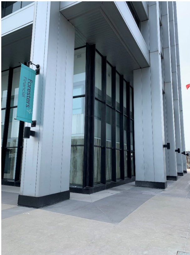
Figure 31. View of the north side of the raised plaza, looking west, showing the double-height curtain wall glazing at the first storey and the piers (Heritage Planning, 2023)
