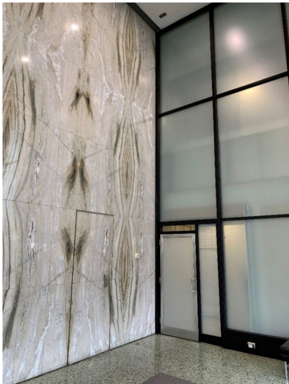
Figure 42. Inside the lobby of the Foresters tower, on the east side of the elevator core, looking north showing the book-matched marble wall panels with the hidden door (Heritage Planning, 2023)
