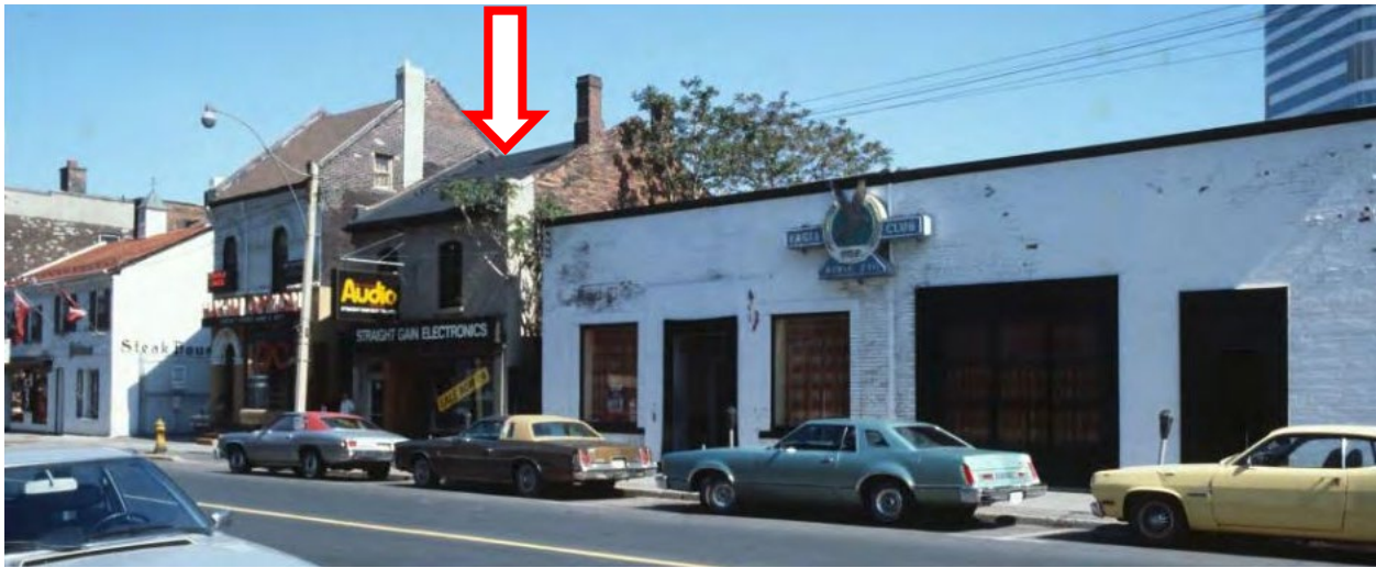
Image 6. 1978-1980 archival photo looking southeast and showing the subject property at centre with other 19th-century properties at left and the 1920s property at 17 Elm at right. (City of Toronto Archives)
